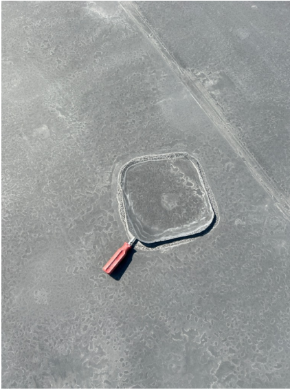
Repair open old repair on Epdm member.
