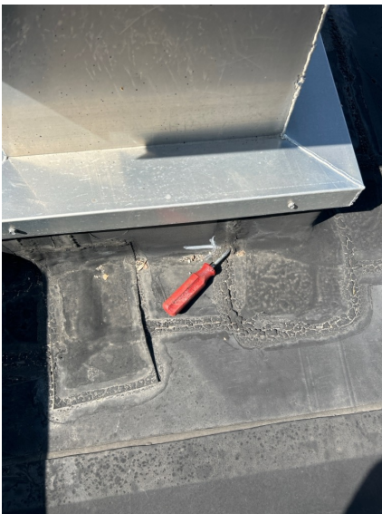
Repair open vent curb flashing.
