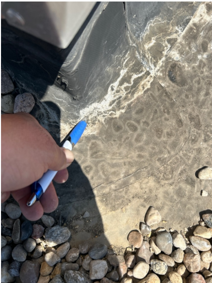
Repair weak power vent curb flashing.
