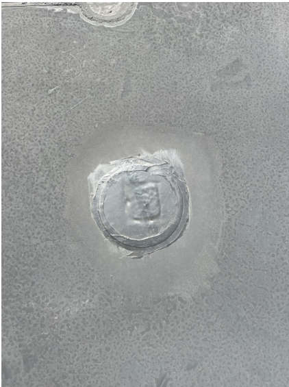
Reinforce 2 thin core cut repairs.
