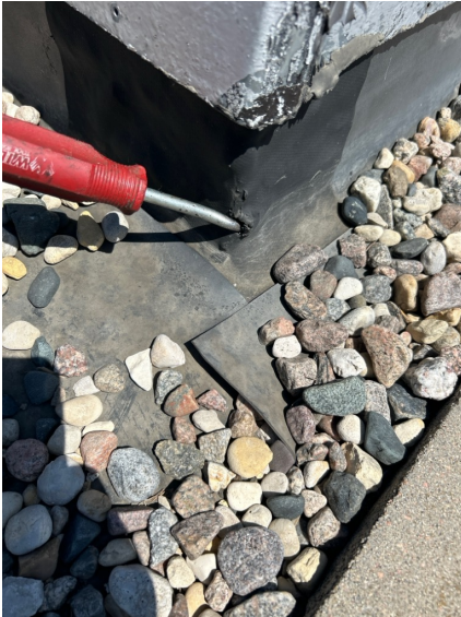
Repair hole in roof hatch curb corner.
