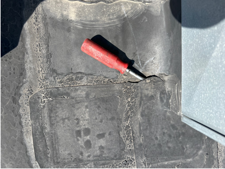
(62) Repair open power vent curb flashing.
