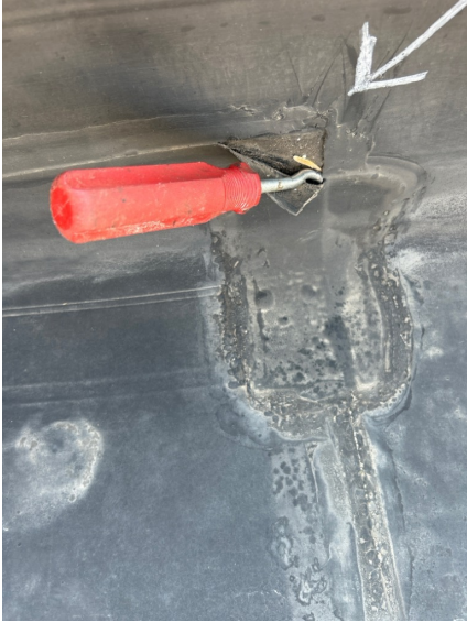
Repair open wall lap flashing.
