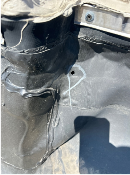
Repair hole in Epdm flashing.
