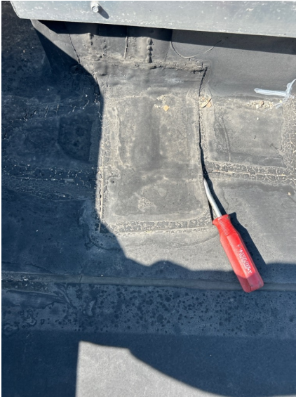
Repair open vent curb flashing.
