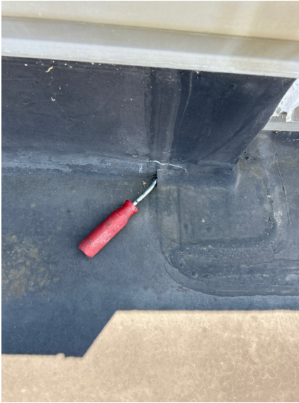
Repair open wall lap flashing.
