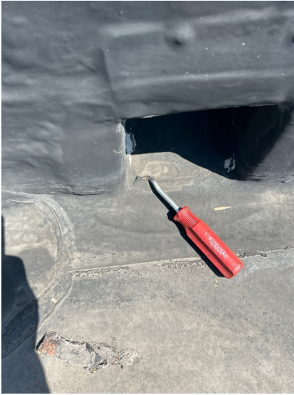
Repair open scupper flashing.
