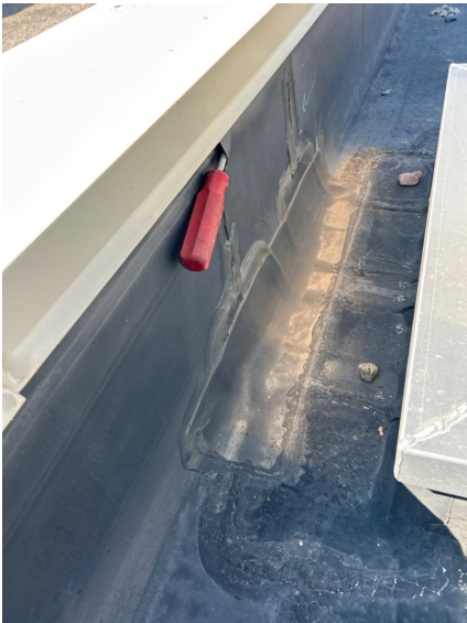
Repair open wall lap flashing.
