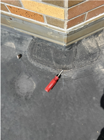
Repair open wall corner flashing.
