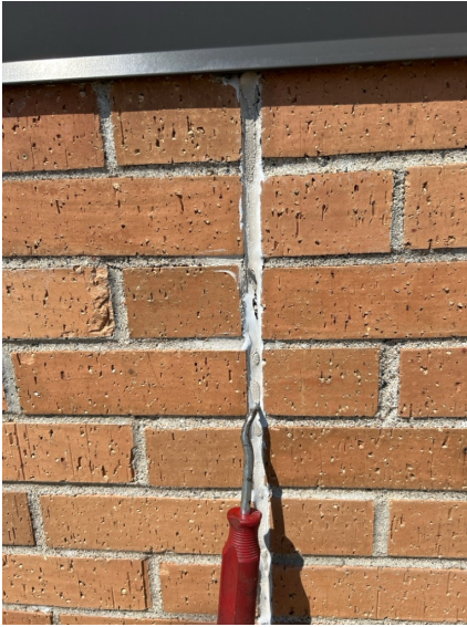
Cleaning and seal 1- 5' open wall control joint.
