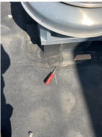
Repair open power vent curb flashing.
