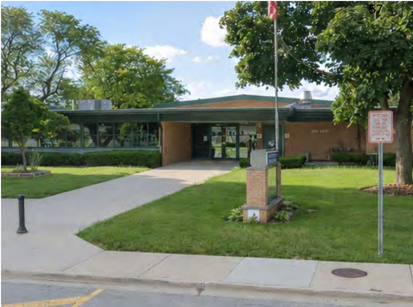
Existing Main Entry
