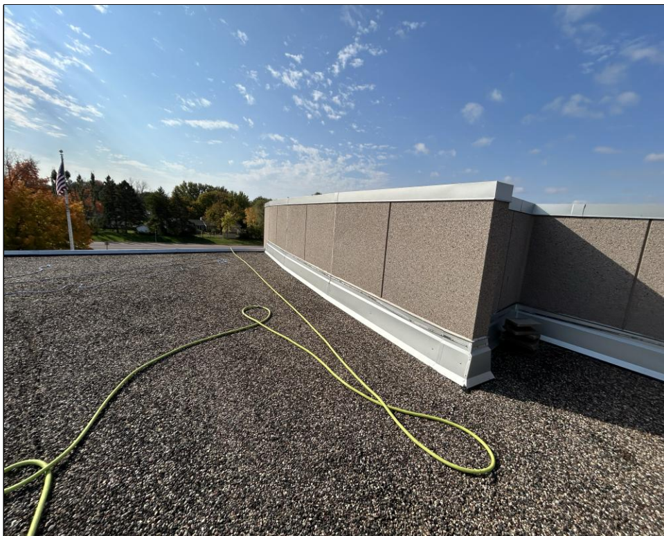
Additional repair location overview.
