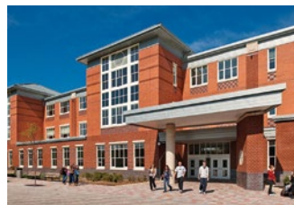
Hanover High School MERV 13 Green Building Design
