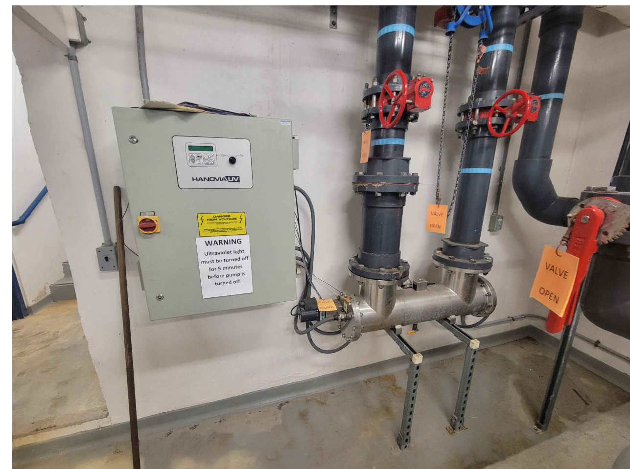
4 EXISTING UV CHAMBER & CABINET AQ0.2 NTS
