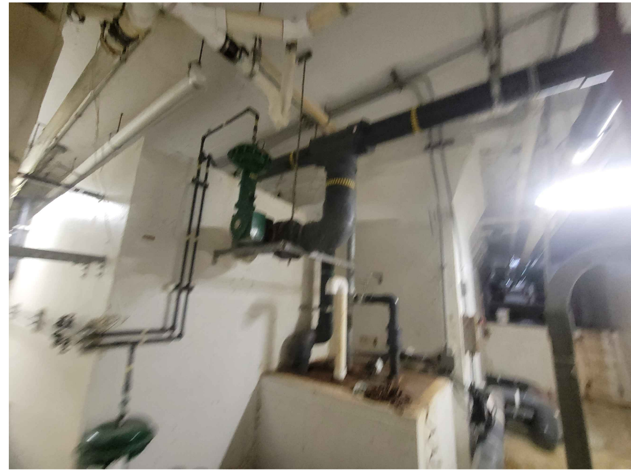
9 AQ0.2 EXISTING GUTTER FISHER VALVE NTS
