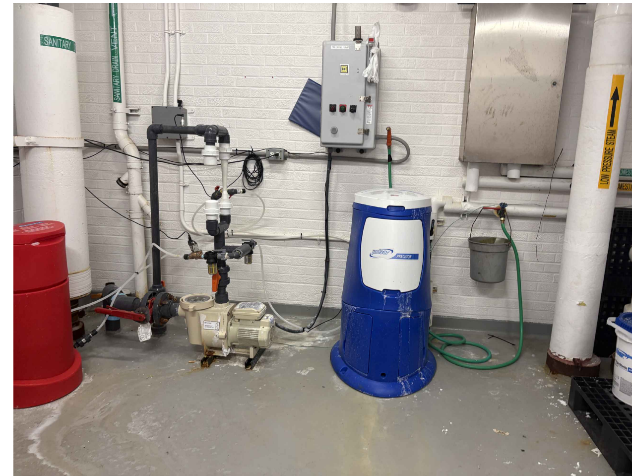
4 AQ0.3 EXISTING CHLORINATION SYSTEM TO REMAIN NTS
