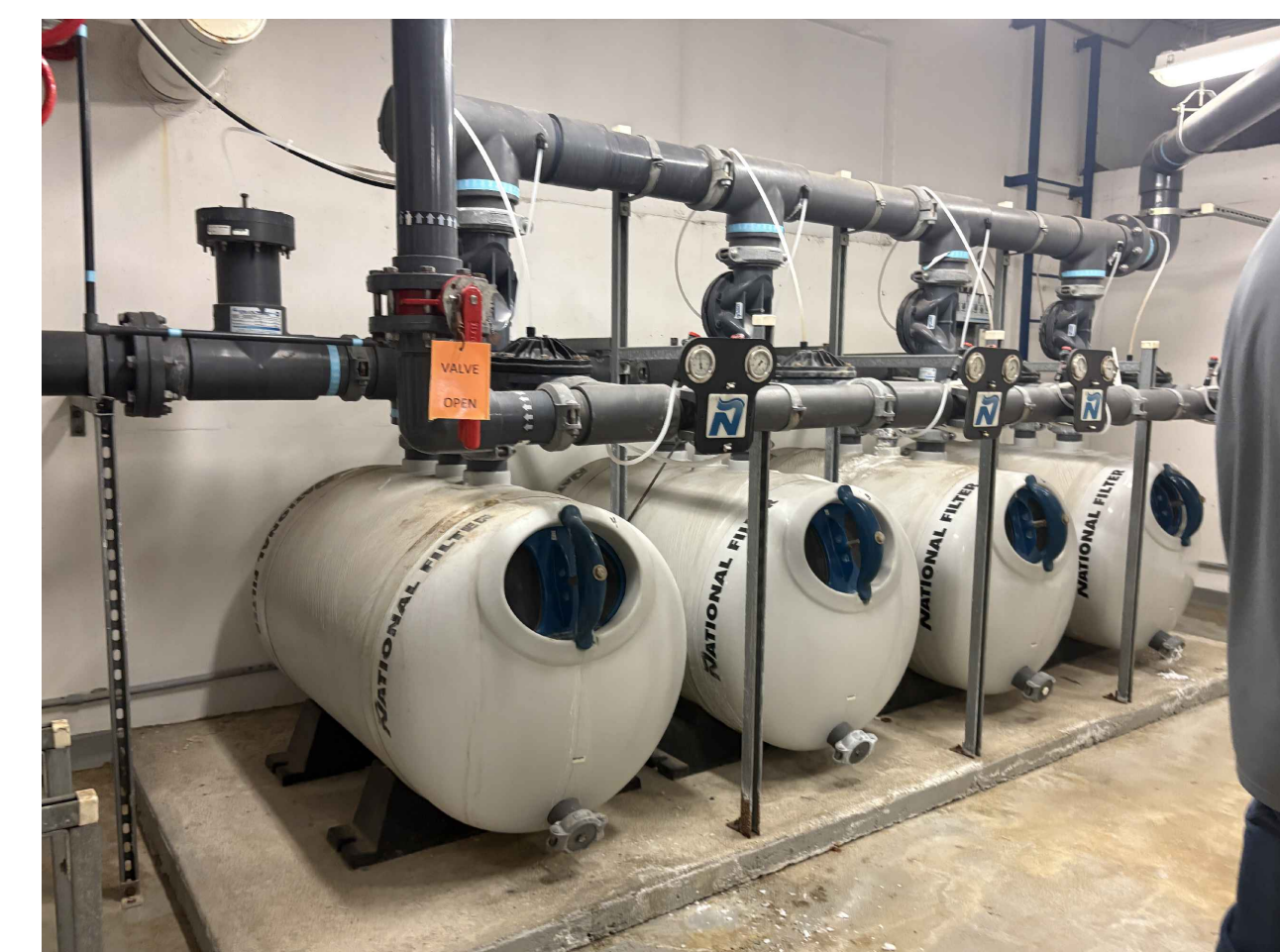
2 EXISTING SAND FILTERS AQ0.2 NTS
