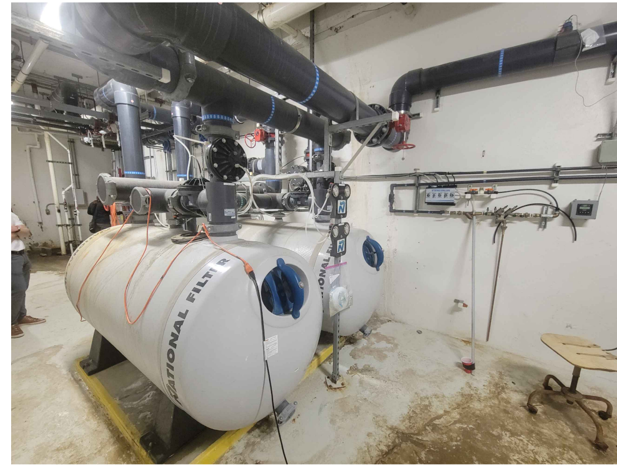
3 AQ0.2 EXISTING SAND FILTERS NTS
