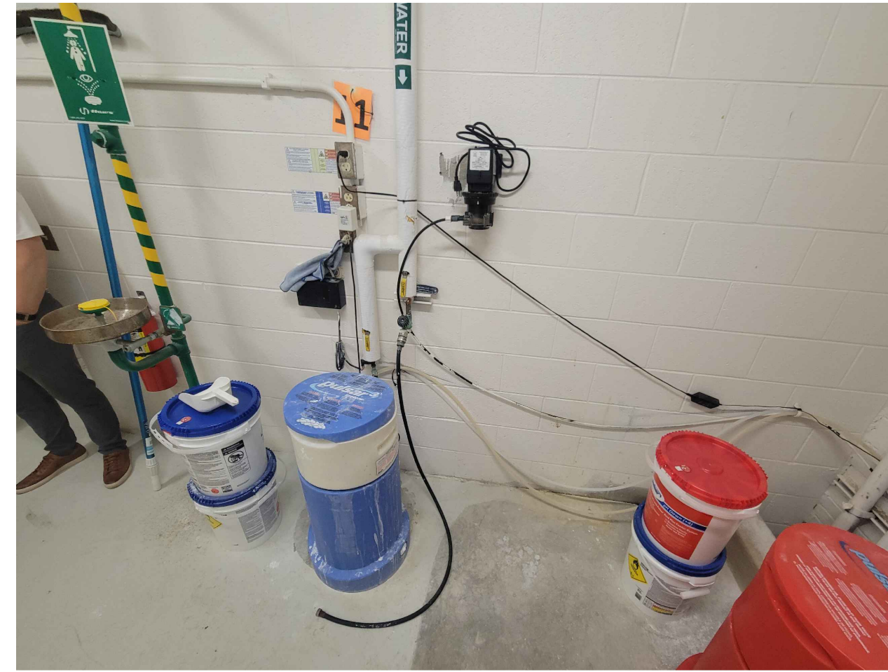
4 AQ0.3 EXISTING CHLORINATION SYSTEM TO REMAIN NTS
