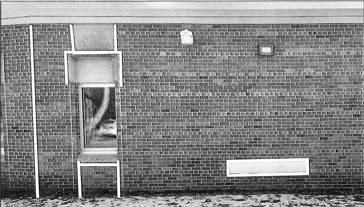
Typical Sealant Replacement
