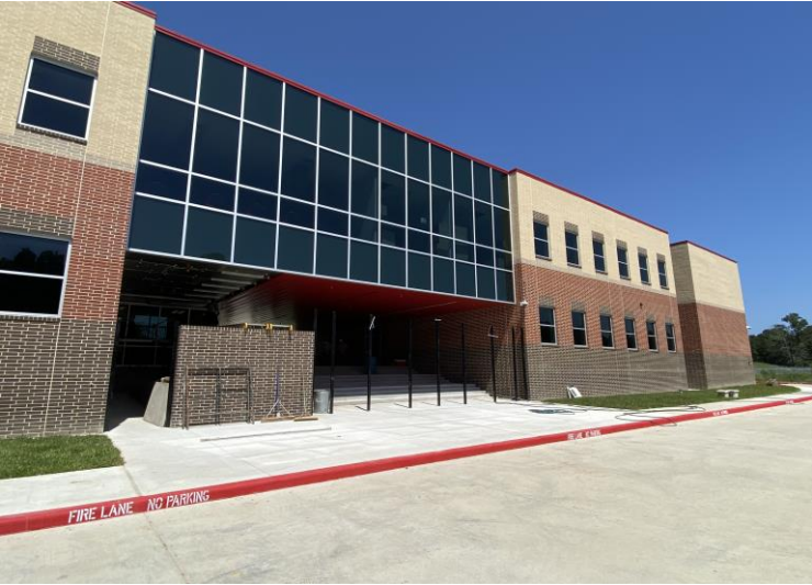
Exterior on the East Side
