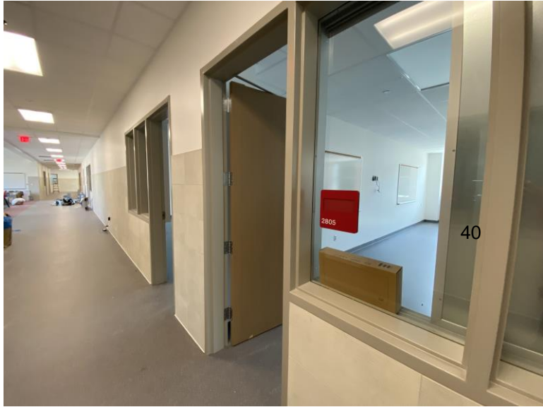
Signage on 2 nd Level
