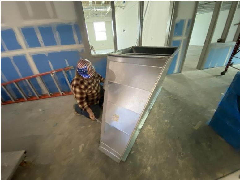
Installing Ductwork on 1 st Level
