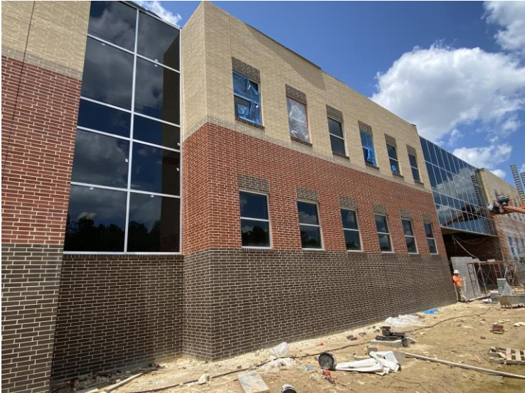
Curtain Walls Installed on the East Side
