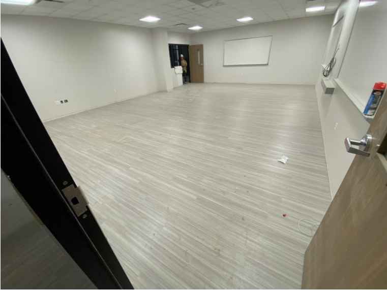
ISS Classroom in Area 2
