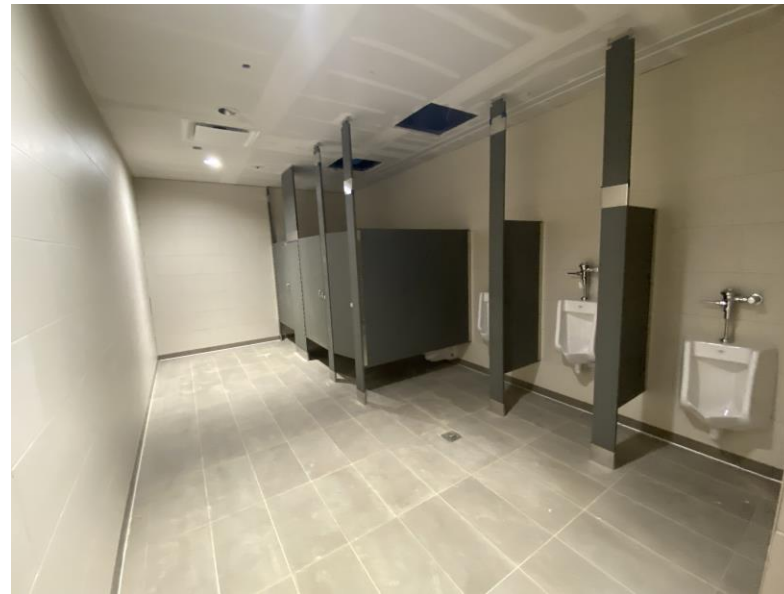
Boys Restroom in Area 3
