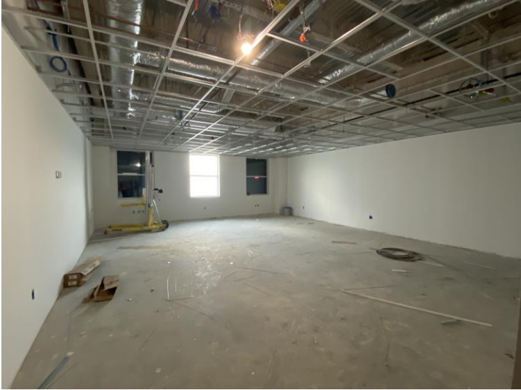
Ceiling Grid Installed on 2 nd Level
