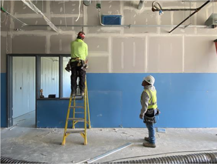
Installing Drywall Joints on 1 st Level
