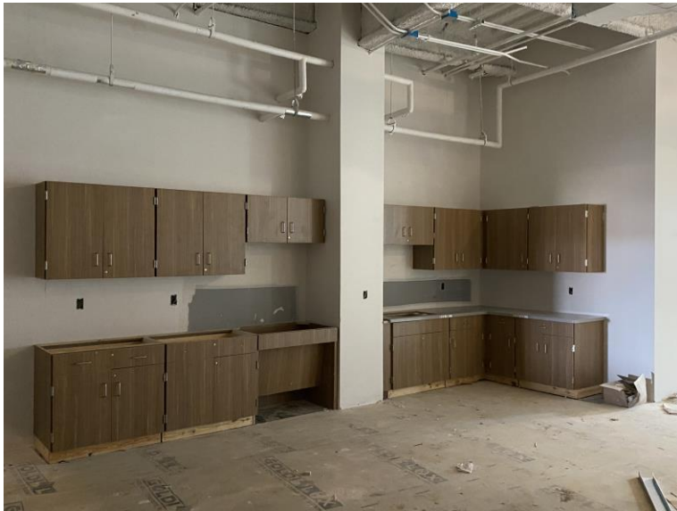
Art Room Millwork in Area 3
