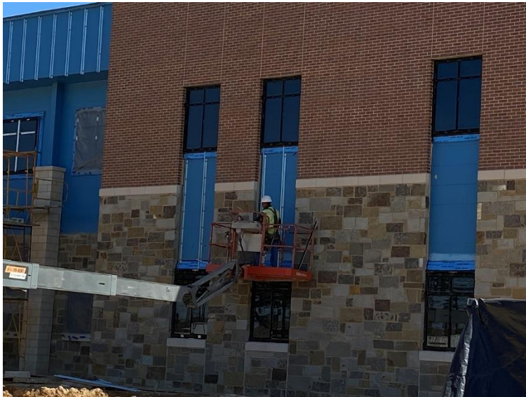
Prepping for Metal Panel in Areas 1 & 8
