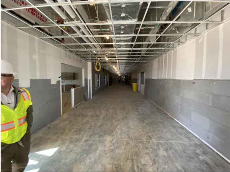
Tile in Corridor in Area 3
