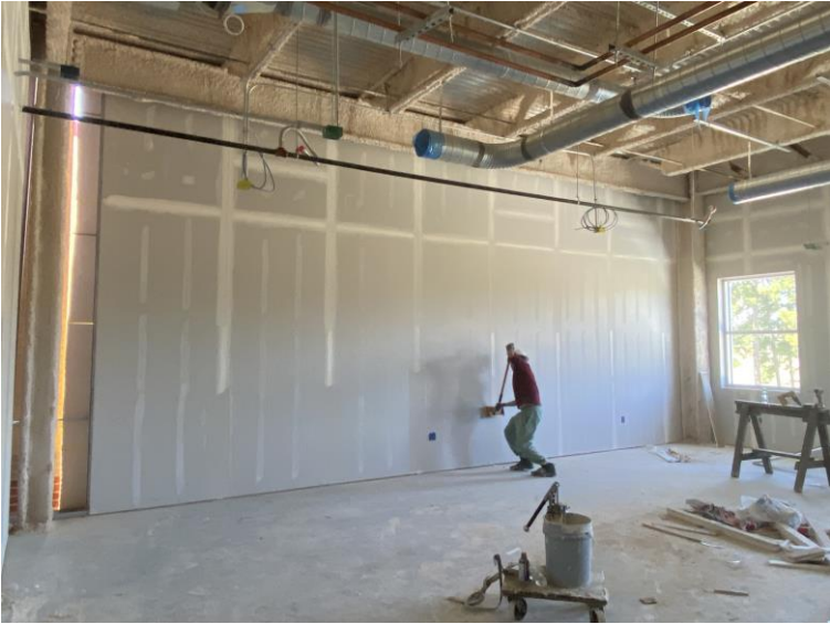
Finishing Drywall on 2 nd Level
