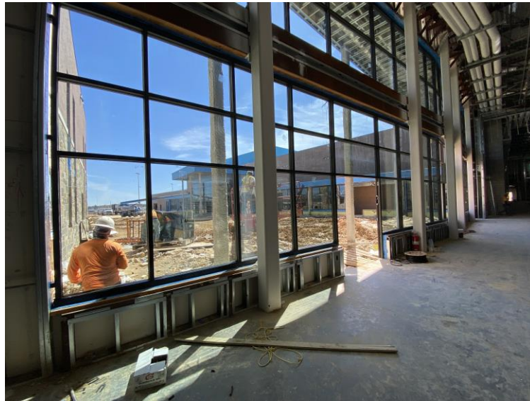
Installing Storefront in Area 3
