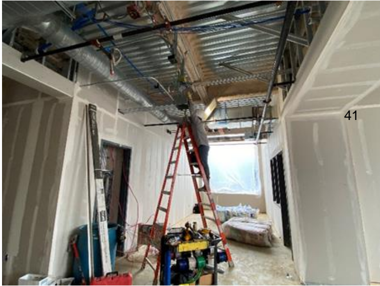
Installing Overhead MEP on 1 st Level
