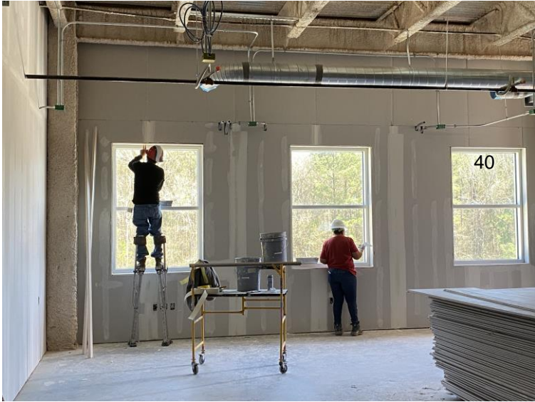
Finishing Windows on 2 nd Level
