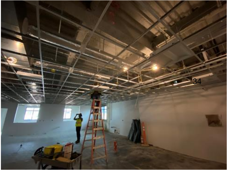
Installing Light Fixtures in Area 1
