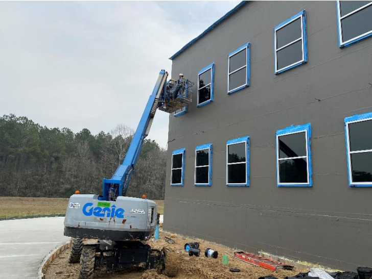
Installing Exterior Windows
