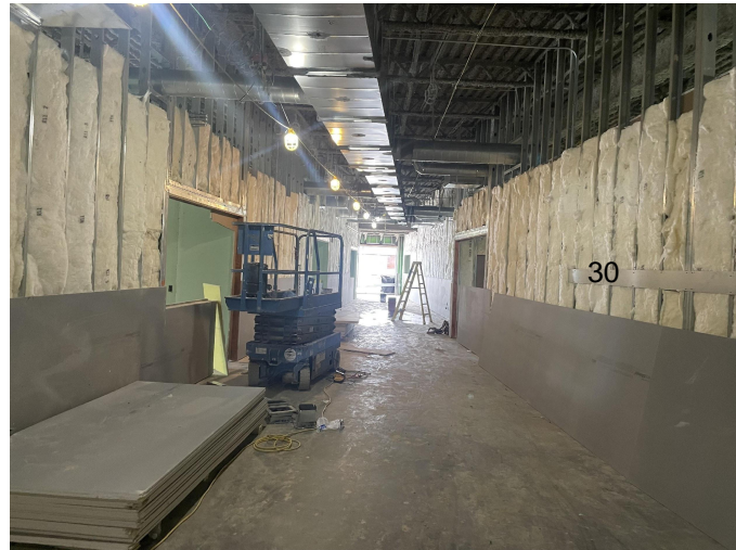
2-side drywall in Area A
