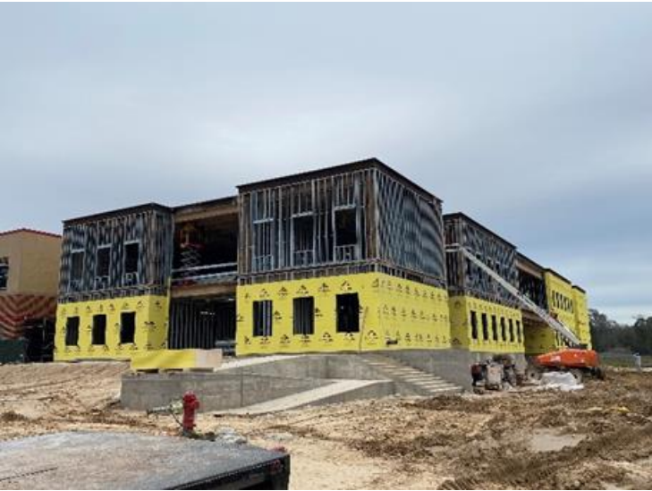
Exterior Sheathing Progress
