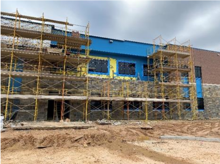
Exterior Brick & Stone in Area 2 & 9
