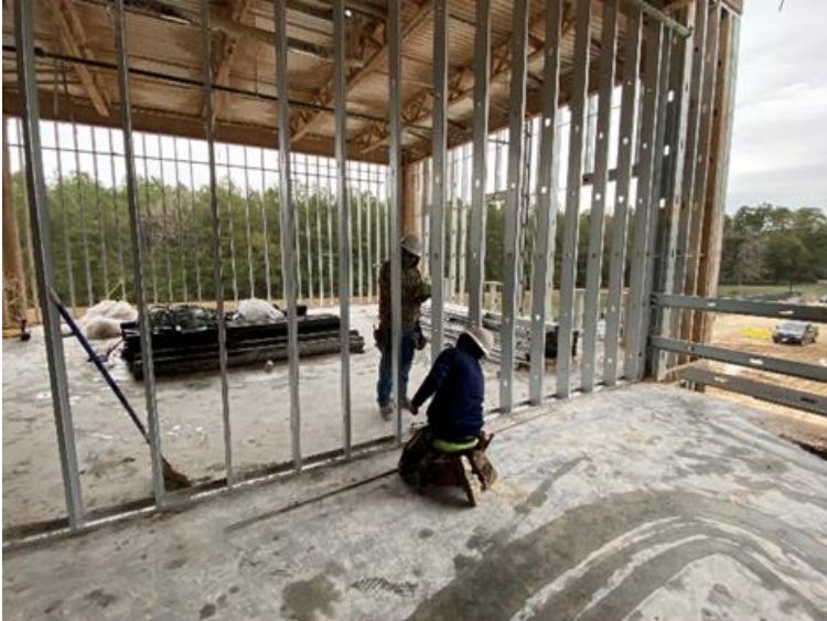
Framing Being Installed on 2 nd Level
