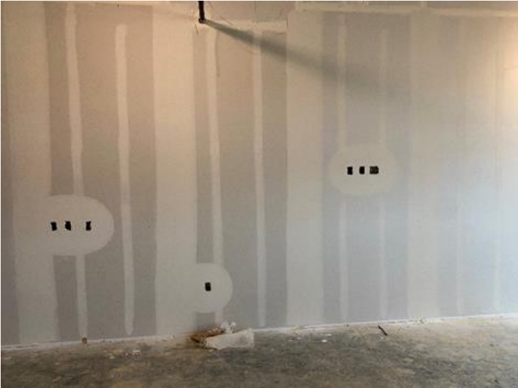
Tape & Float in Area 2
