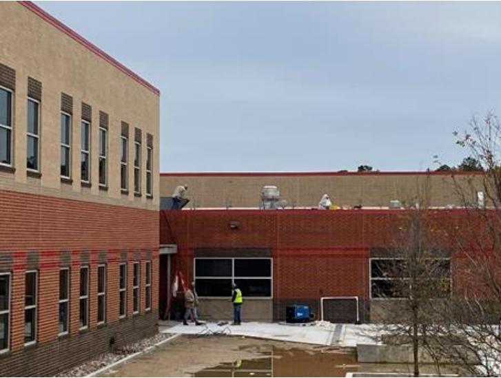
Mechanical Work in Existing Campus
