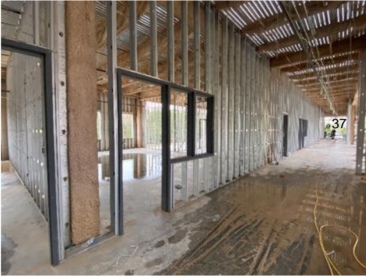
Interior Frames Installed on 2 nd Level
