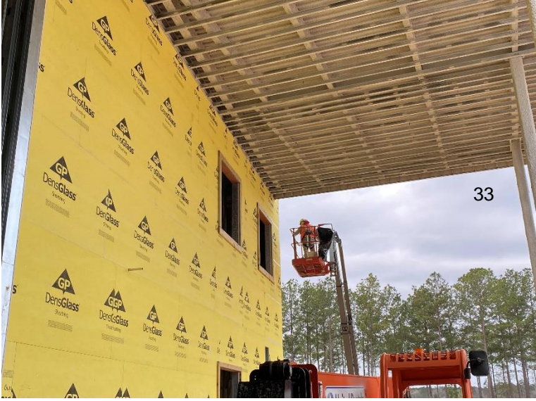
Exterior Sheathing Area 1
