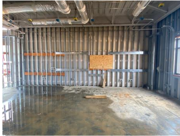
Backing Installed for Teaching Wall
