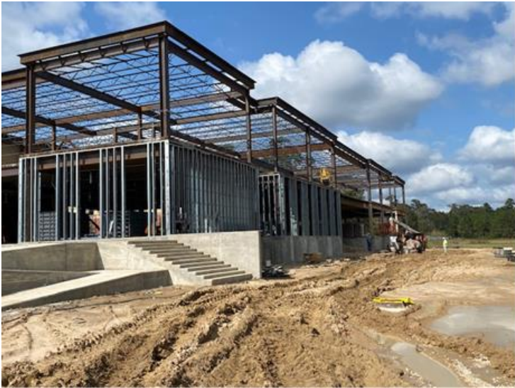
Cold Formed Metal Framing Progress
