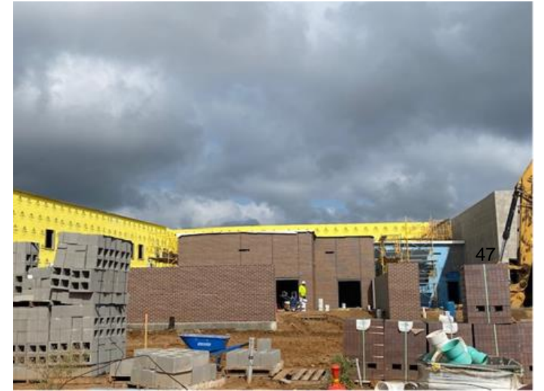
Exterior Brick in Area 4
