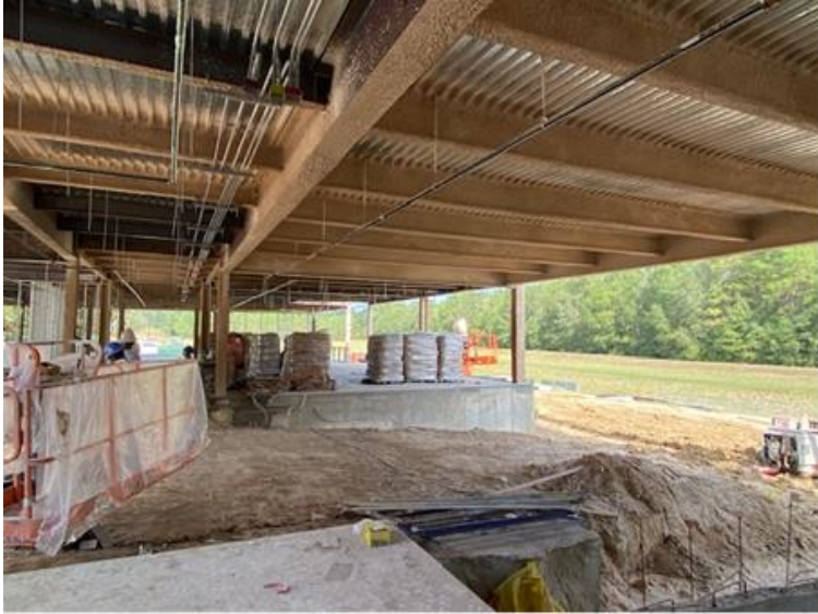
Fireproofing on 1 st Level
