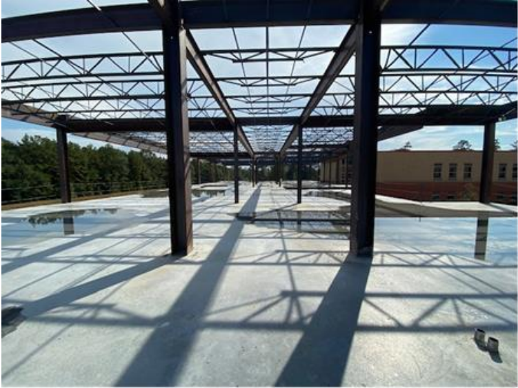
2 nd Level Deck Poured
