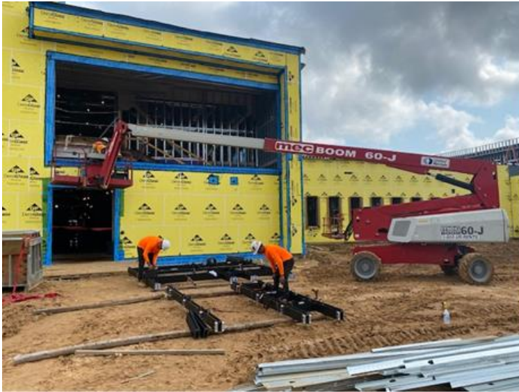
Installing Exterior Window Frame
