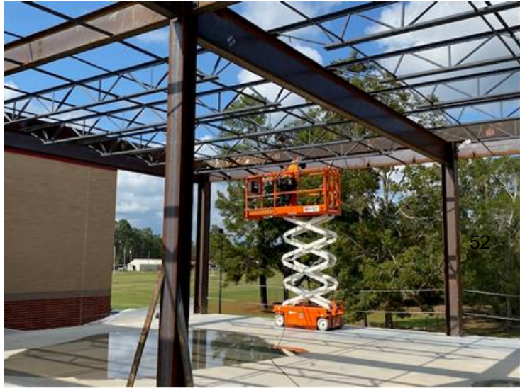
Welding Bolts on 2 nd Level
