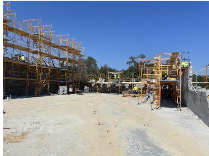
CMU in Area E
