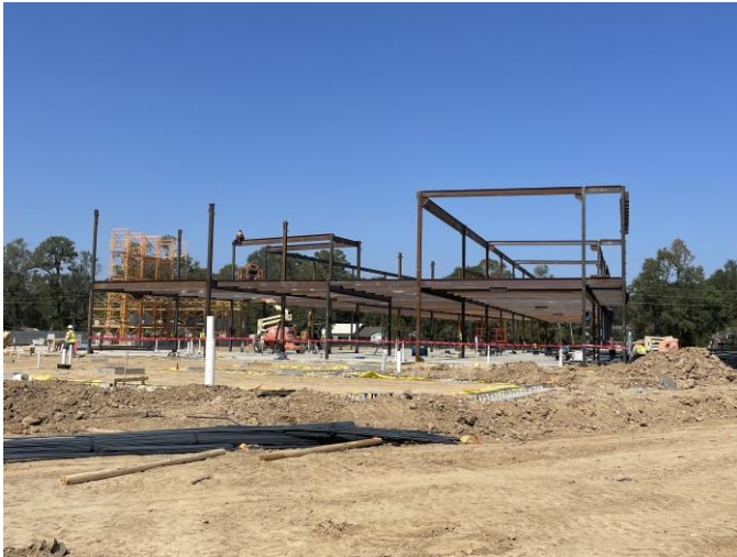
Steel Erection in Area C
