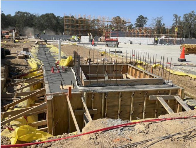
Elevator pit and grade beams
