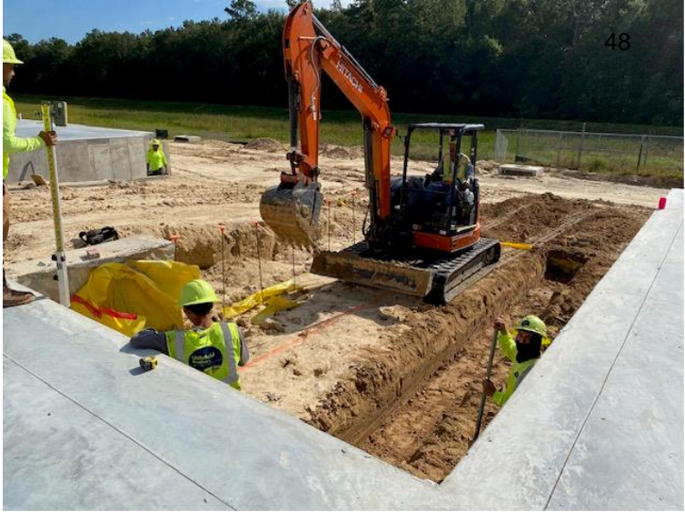
Trenching for Ramp Footings
