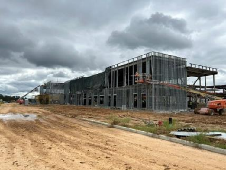
Metal Framing Going Up in Area 9 & 2
