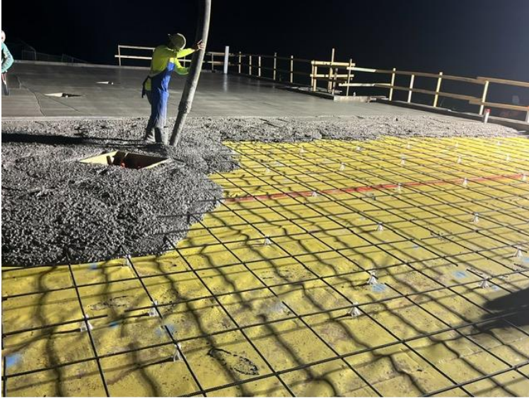
Pouring Slab on Grade
