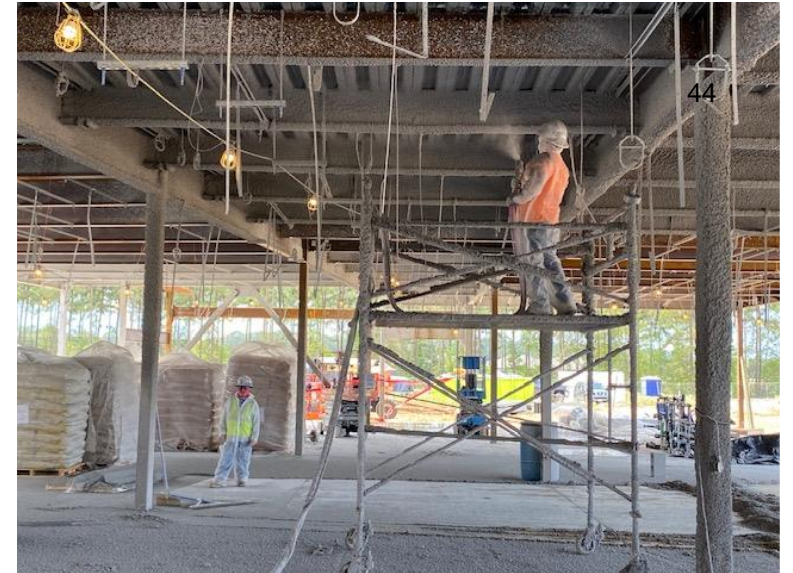
Installing Overhead Fireproofing
