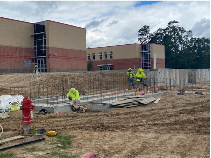
Footings for ADA Ramp & Stairs
