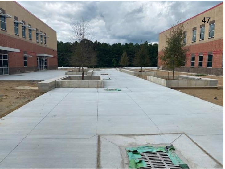
Courtyard Flatwork Installed
