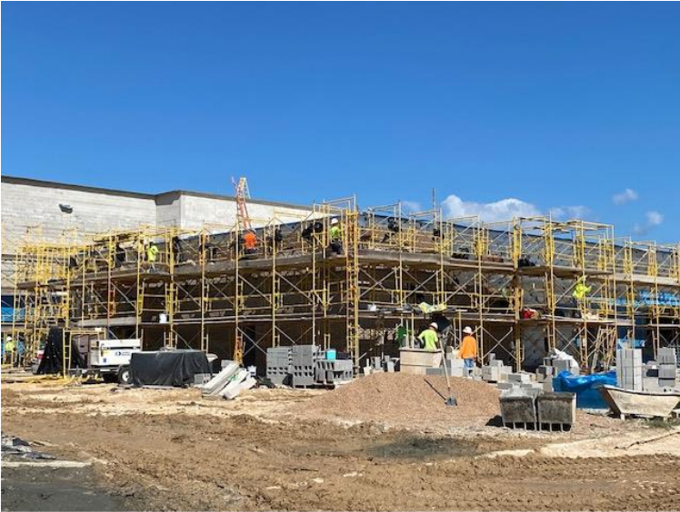
Installing Exterior Brick in Area 7
