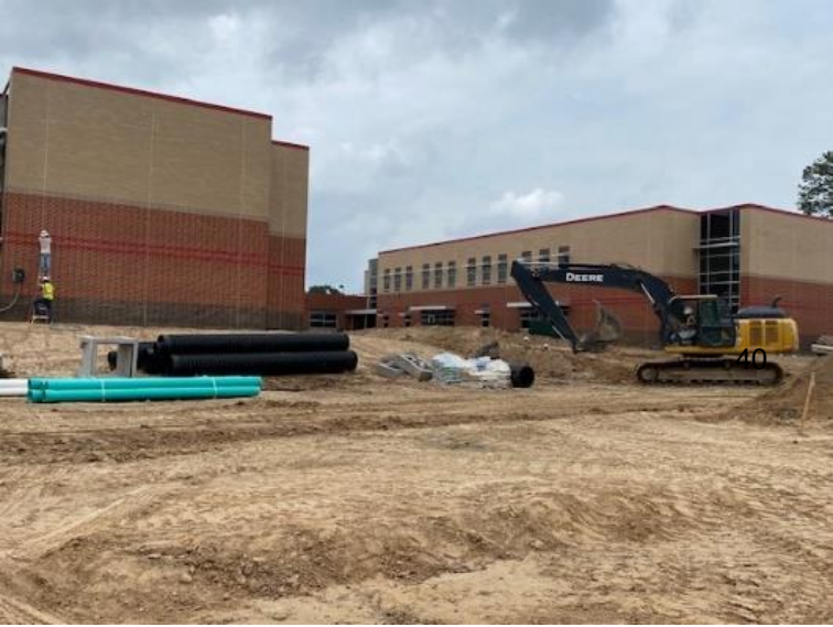
Staging of Underground Utility Pipes
