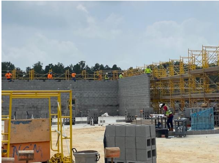
Installing CMU Wall Partitions
