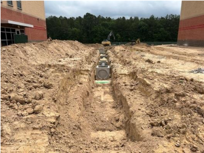
Storm Sewer Installation in Courtyard
