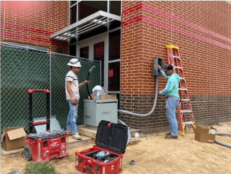
Installing Temporary Power
