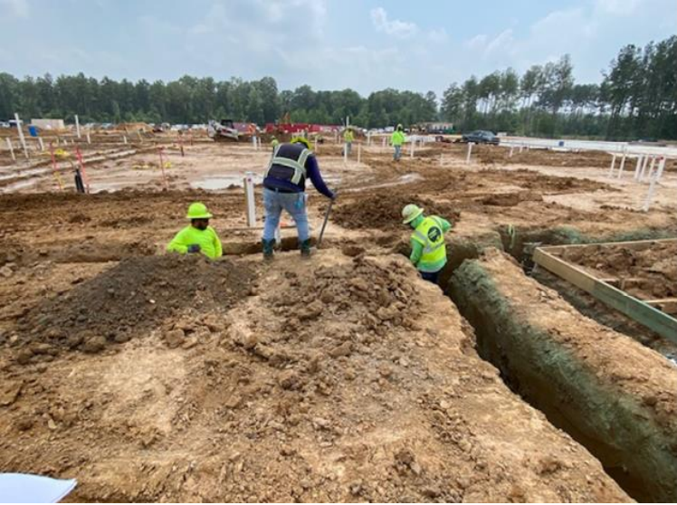
Digging Trenches for Grade Beam
