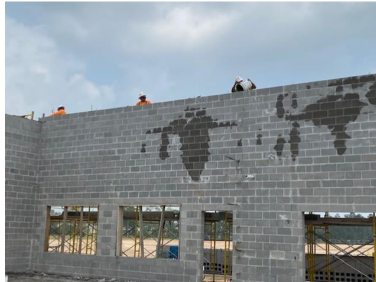
Placing Grout in CMU
