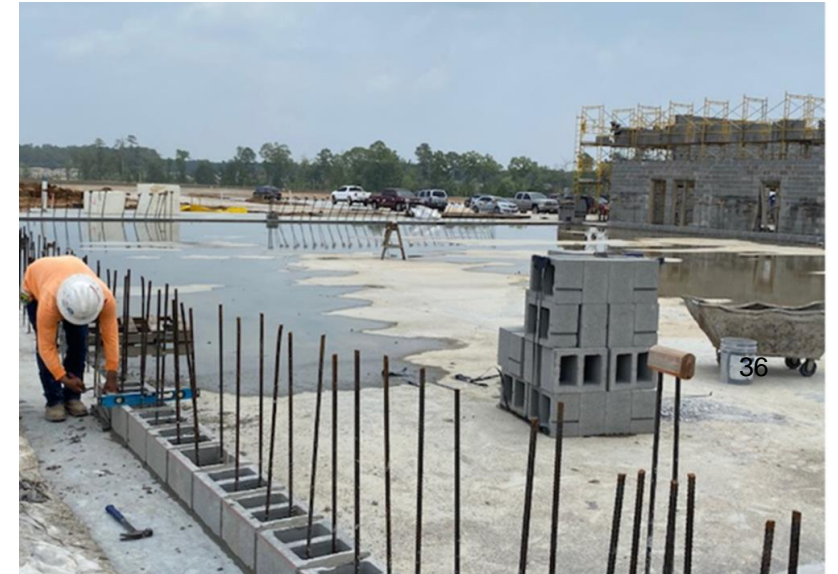
Leveling Large CMU in Gym Area
