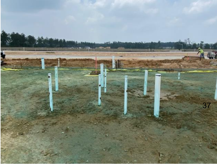
Plumbing Stub out for Restrooms
