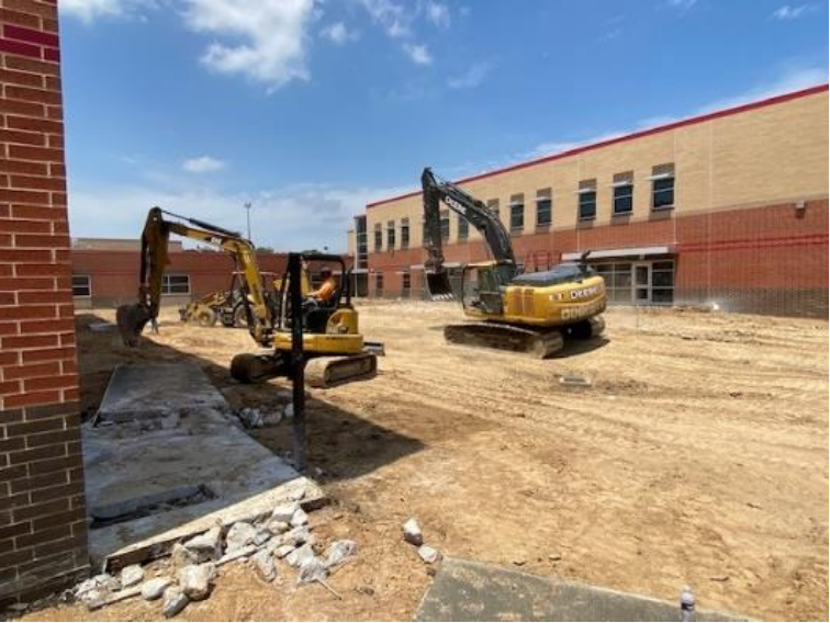
Demolition of Courtyard & Sidewalk
