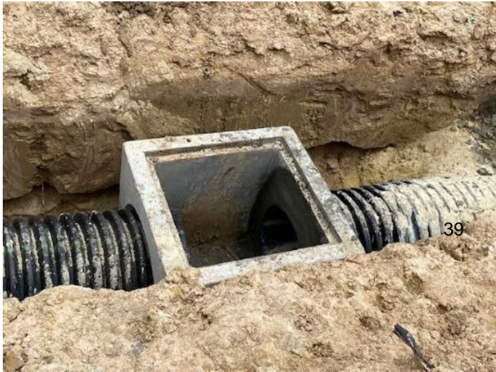
Storm Sewer Manhole
