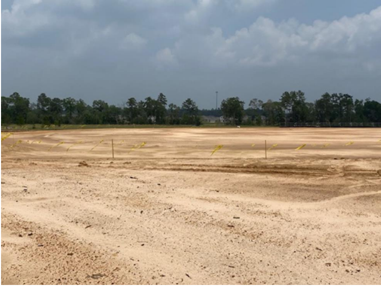
Track & Field Prepped and Flagged Off
