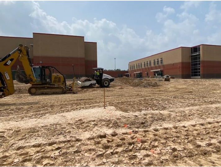
Compacting Roadway Earthwork
