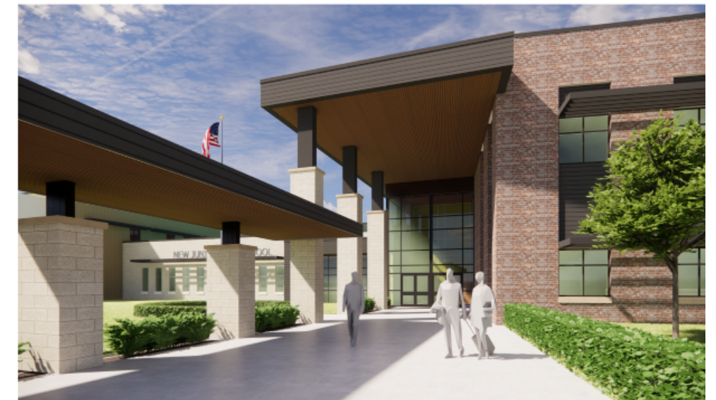
MAIN ENTRY WALKWAY
