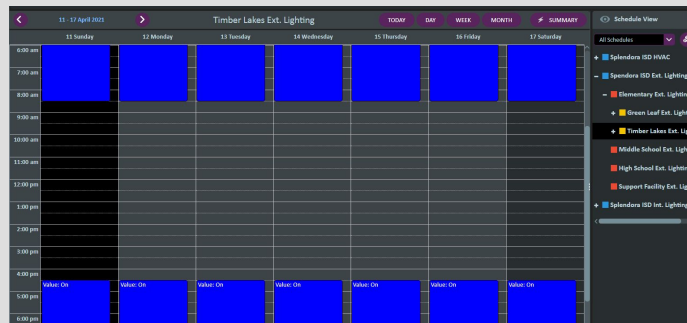
BAS/Controls lighting scheduler
