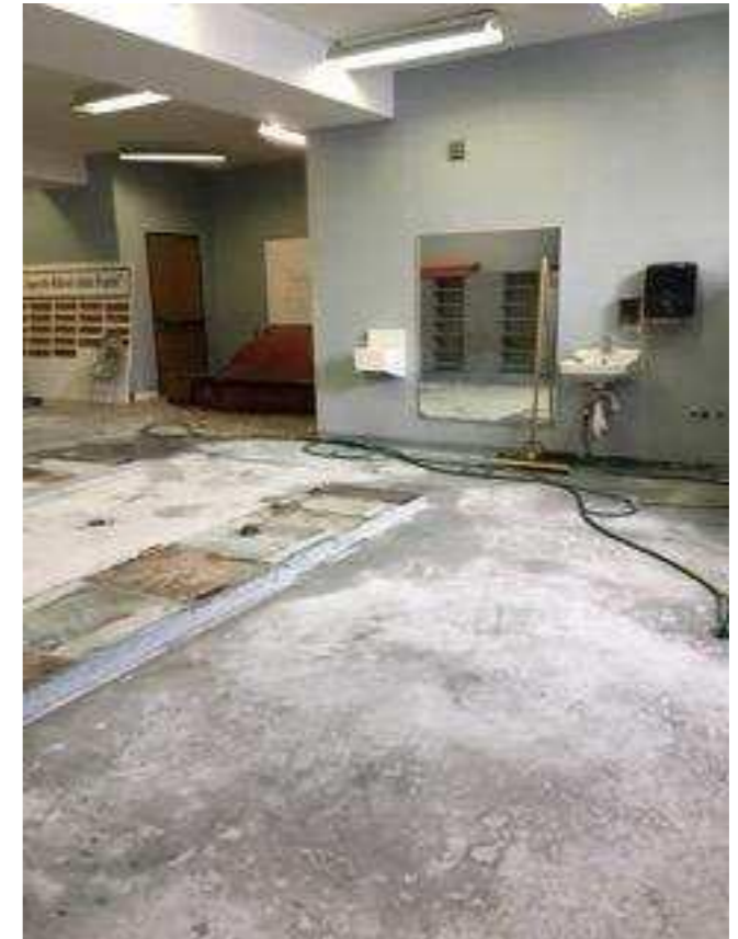
Initial stage of floor paint removal completed
