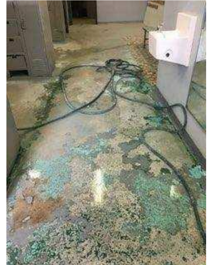
Early stages of floor stripping Note the multiple layers of paint
