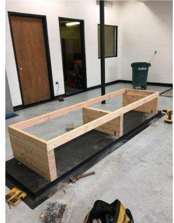
Assembly of first custom bench begins.
