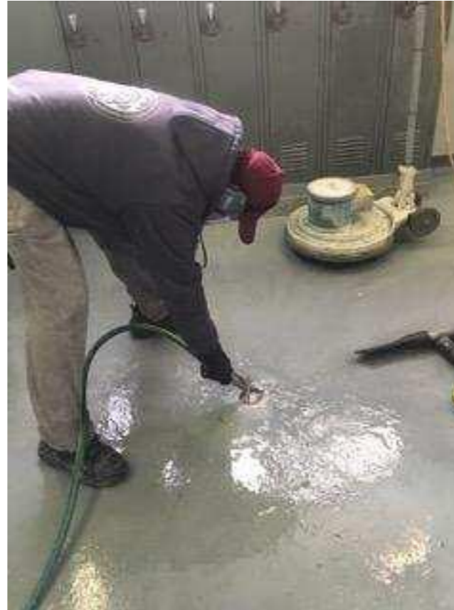
Prepping floor for grinder
