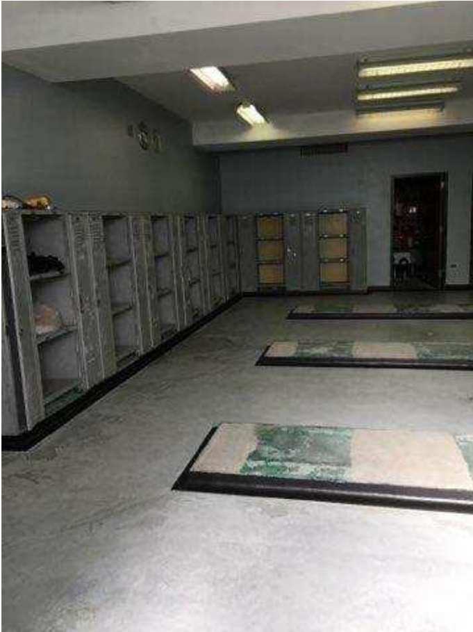
Lockers and walls prepped for paint
