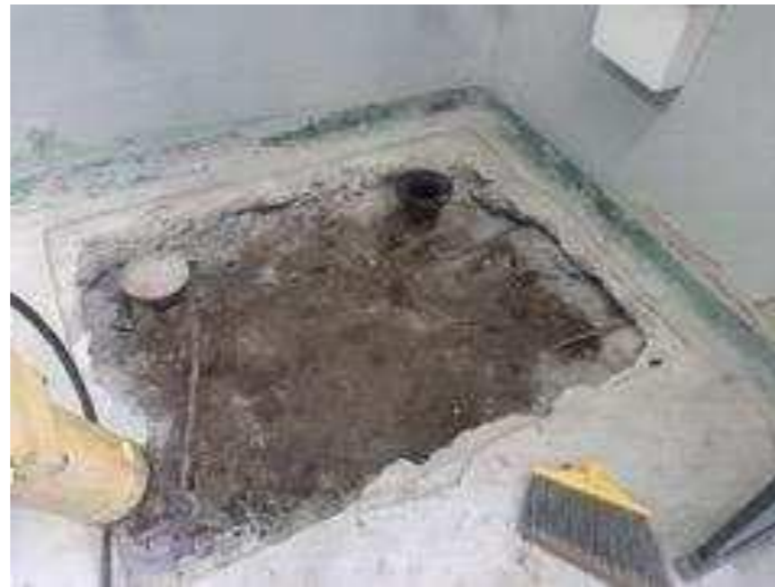
Concrete and underground plumbing repair
