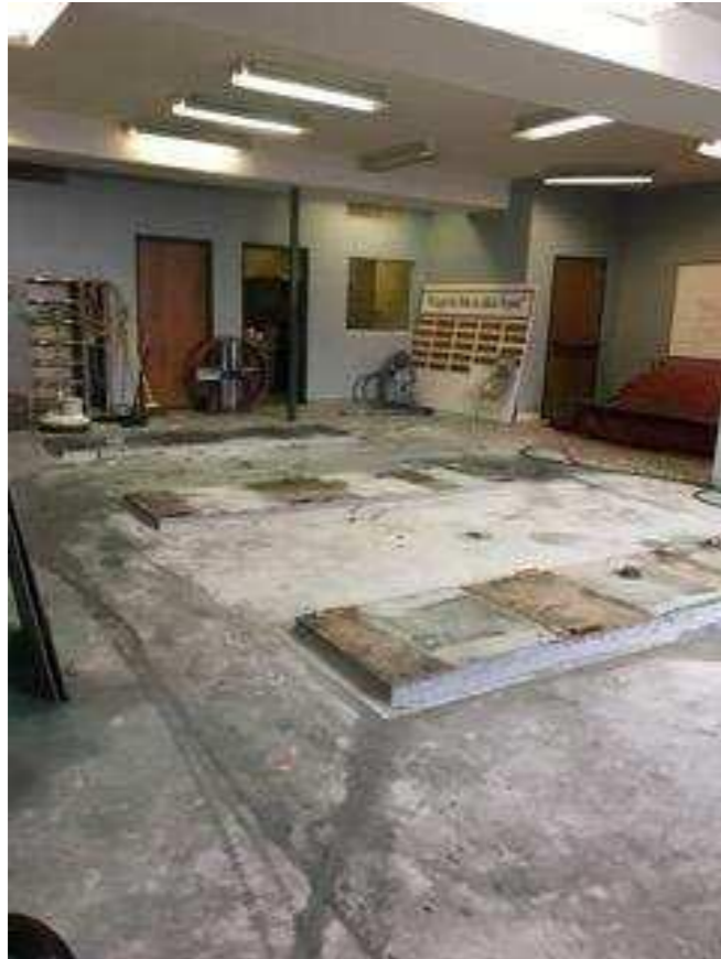
Center lockers removed
