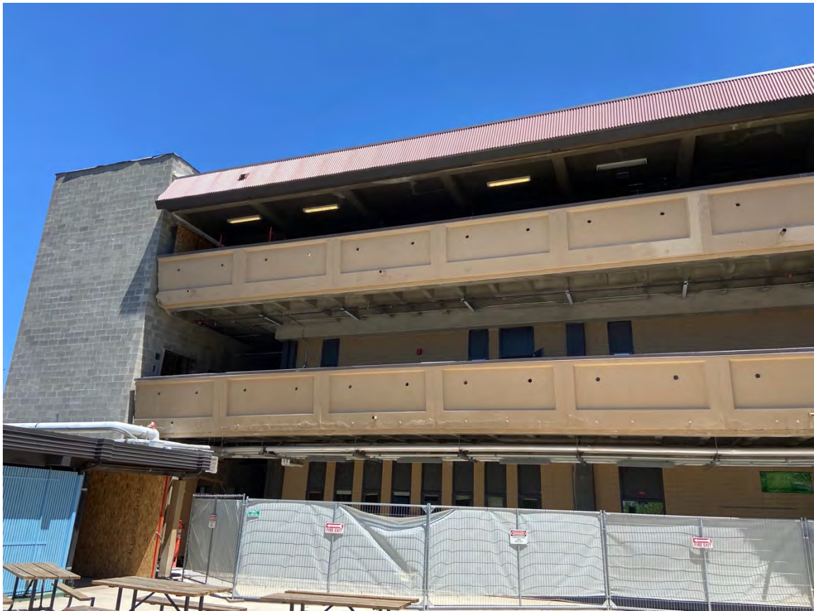
AHS Humanities Building Exterior Prepped for Demo
