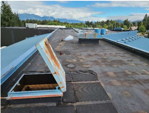
Roof L access hatch
