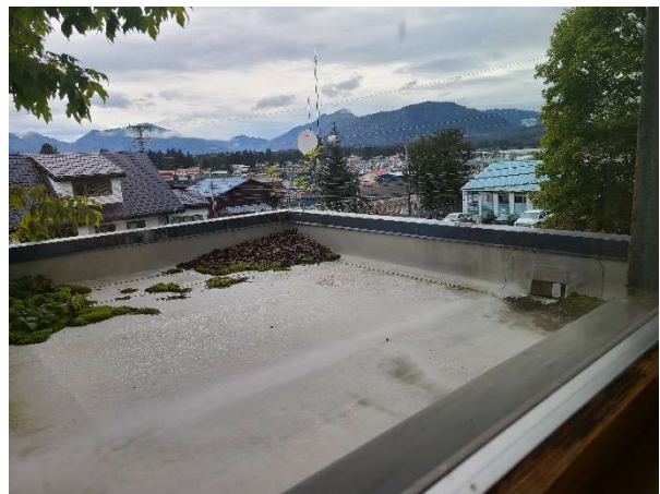
Scupper and vegetation of Roof B
