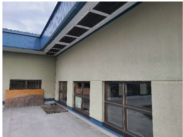
Plywood used to protect windows from ice
