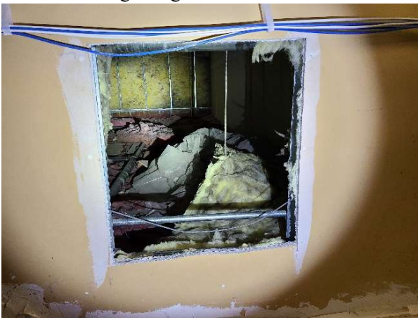
Opening from Mechanical Room into Attic
