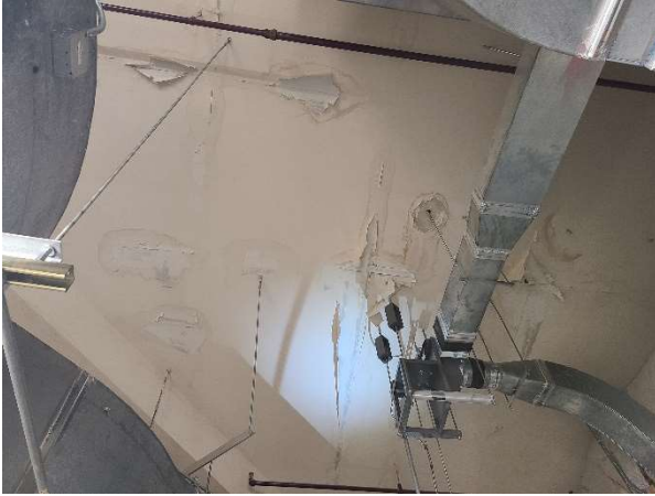
Mechanical room ceiling
