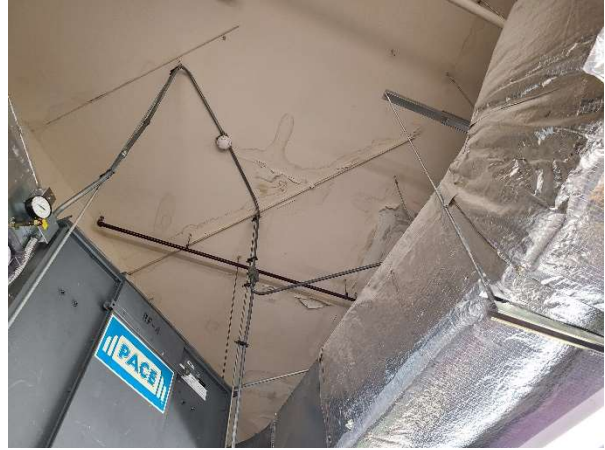
Mechanical room ceiling
