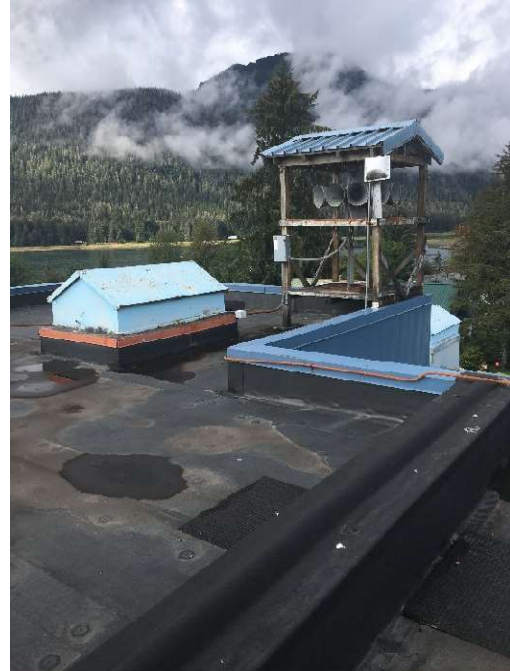
Stage smoke hood/tsunami warning
