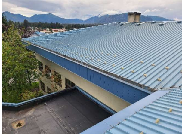
Roof C shedding onto Roof N
