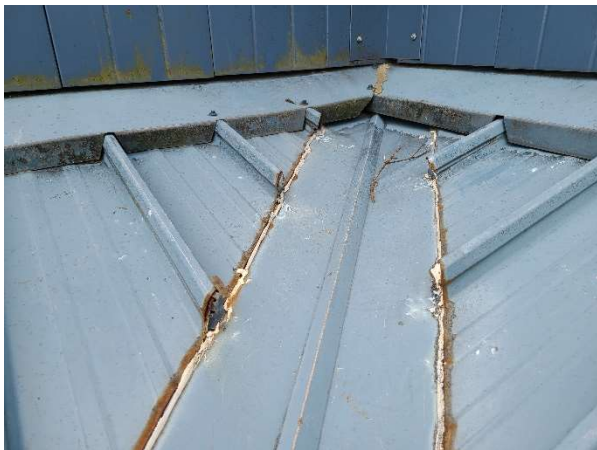
Metal roof valley
