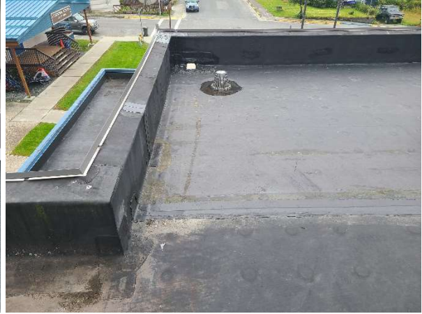
2022 partial membrane repair
