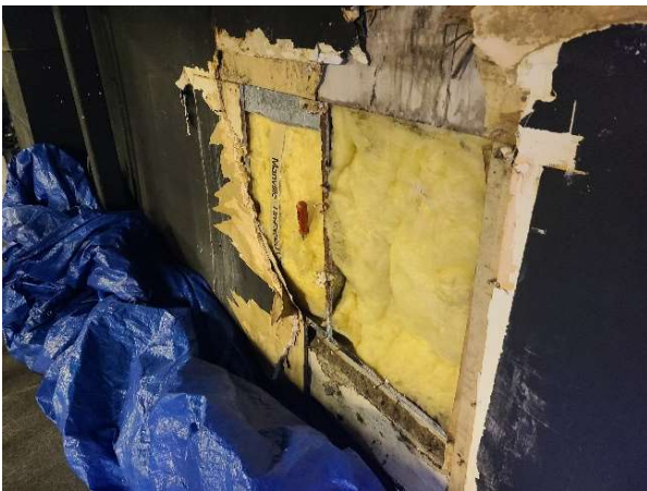
Opening cut into the wall
