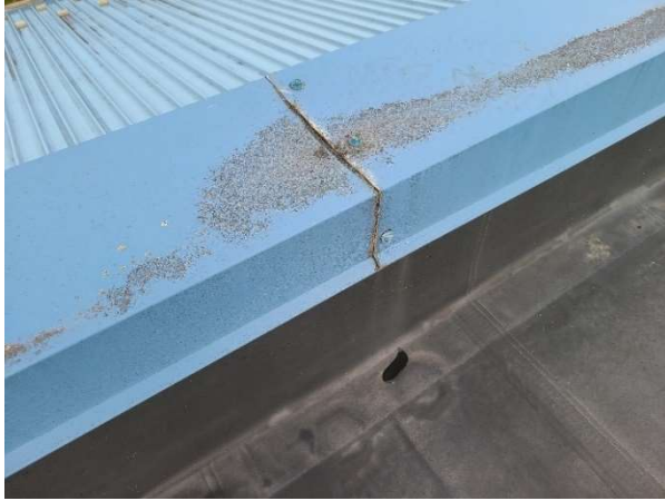
Parapet cap installation
