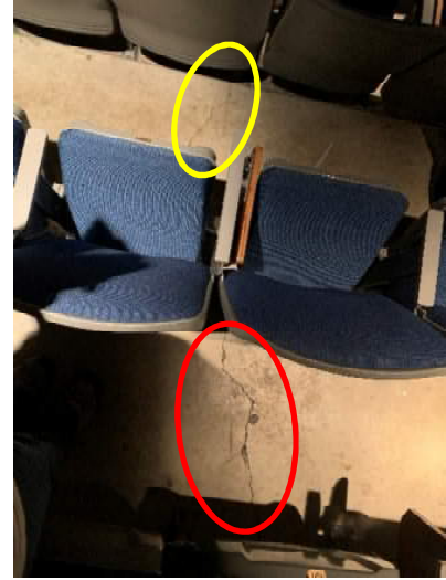
Figure 3- 2020 Riser Cracks
