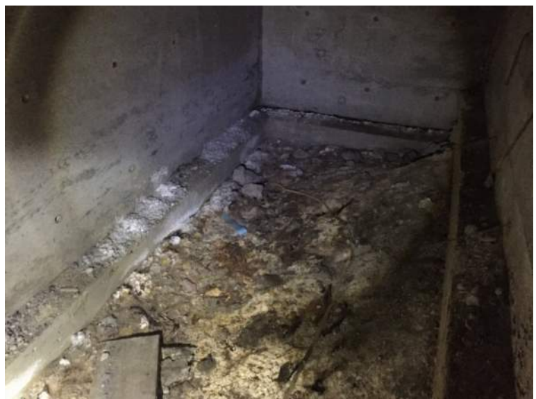
Figure 13- Exposed Footings
