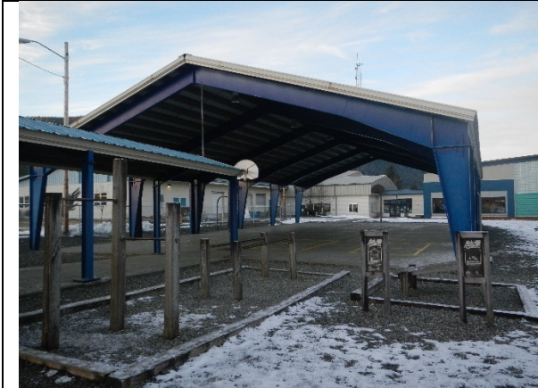
Covered Play Area. (Photo DEED 2016 Archive.)
