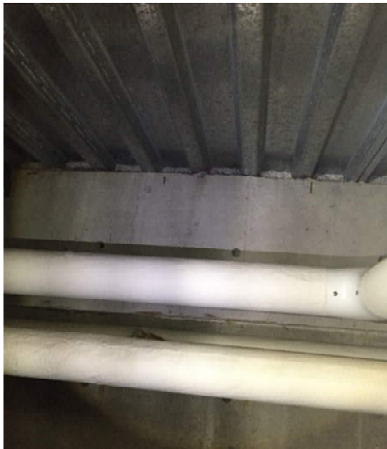
Figure 12- Pan Decking under Floor Slab
