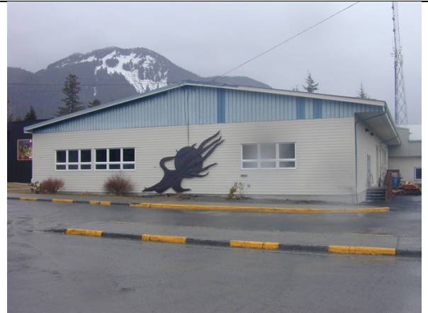
Technical Arts Building. (Photo DEED 2011 Archive.)
