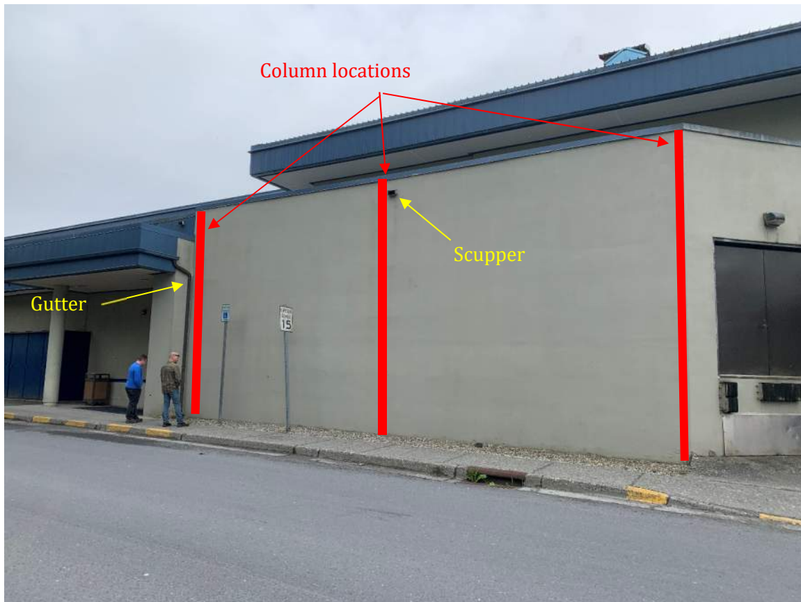
Figure 19- 2020 North Wall of Addition, Column Locations
