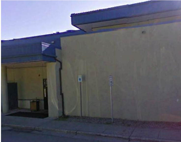
Figure 17- 2018 North Wall of Addition, East and Middle Column Locations
