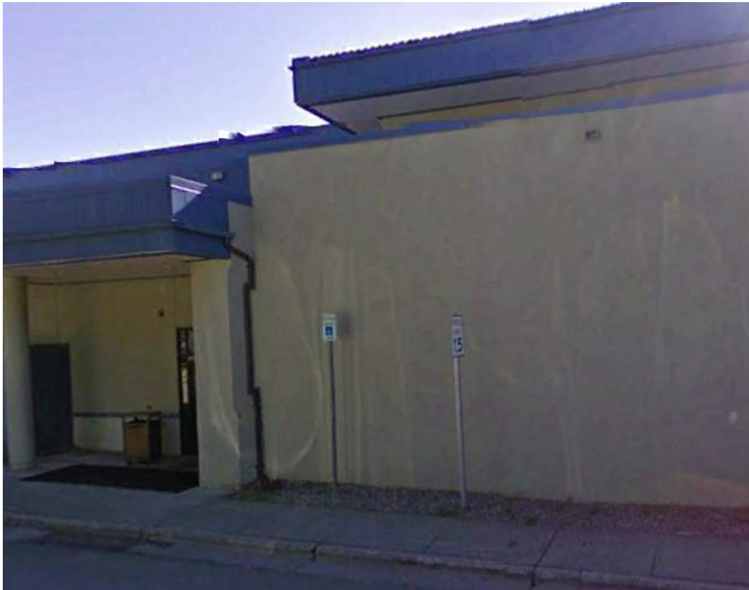
Figure 14- North Wall of Addition, East and Middle Post Locations
