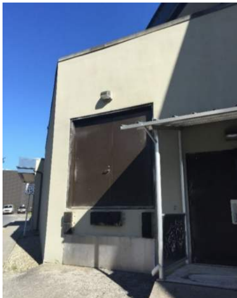
Figure 15- Northwest Wall of Addition, West Post
