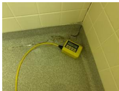
Figure 13- 2020 Boys Bathroom Floor
