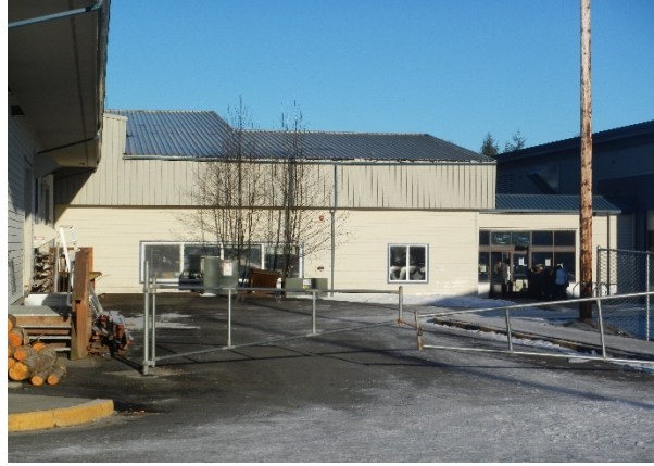
Community Gym / Aquatic Center. (Access point: 1995 Gym on left, 2006 Aquatic Center on right.) (Photo DEED 2016 Archive.)
