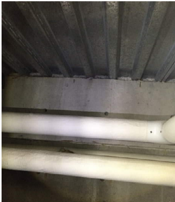
Figure 12- Pan Decking under Floor Slab
