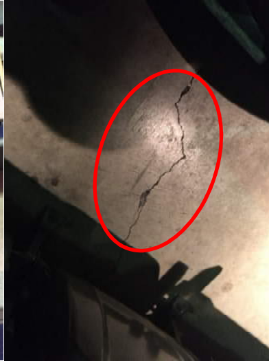
Figure 2- 2018 Riser Crack
