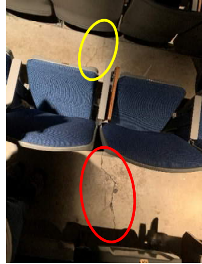
Figure 3- 2020 Riser Cracks
