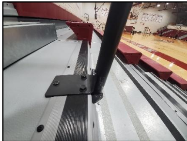
Handrail anchor attachment.
