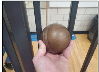
Proper guardrail gap closure.
