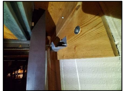
Upper wall anchor attachment.
