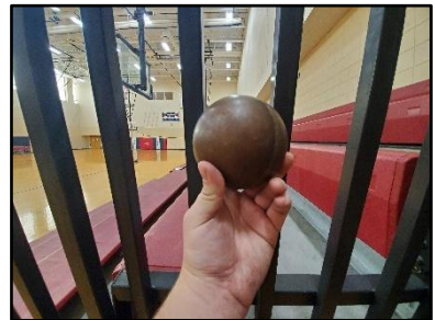
Proper guardrail gap closure.
