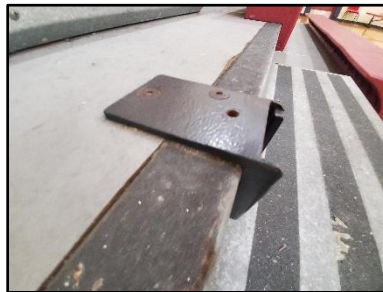
Handrail anchor attachment.
