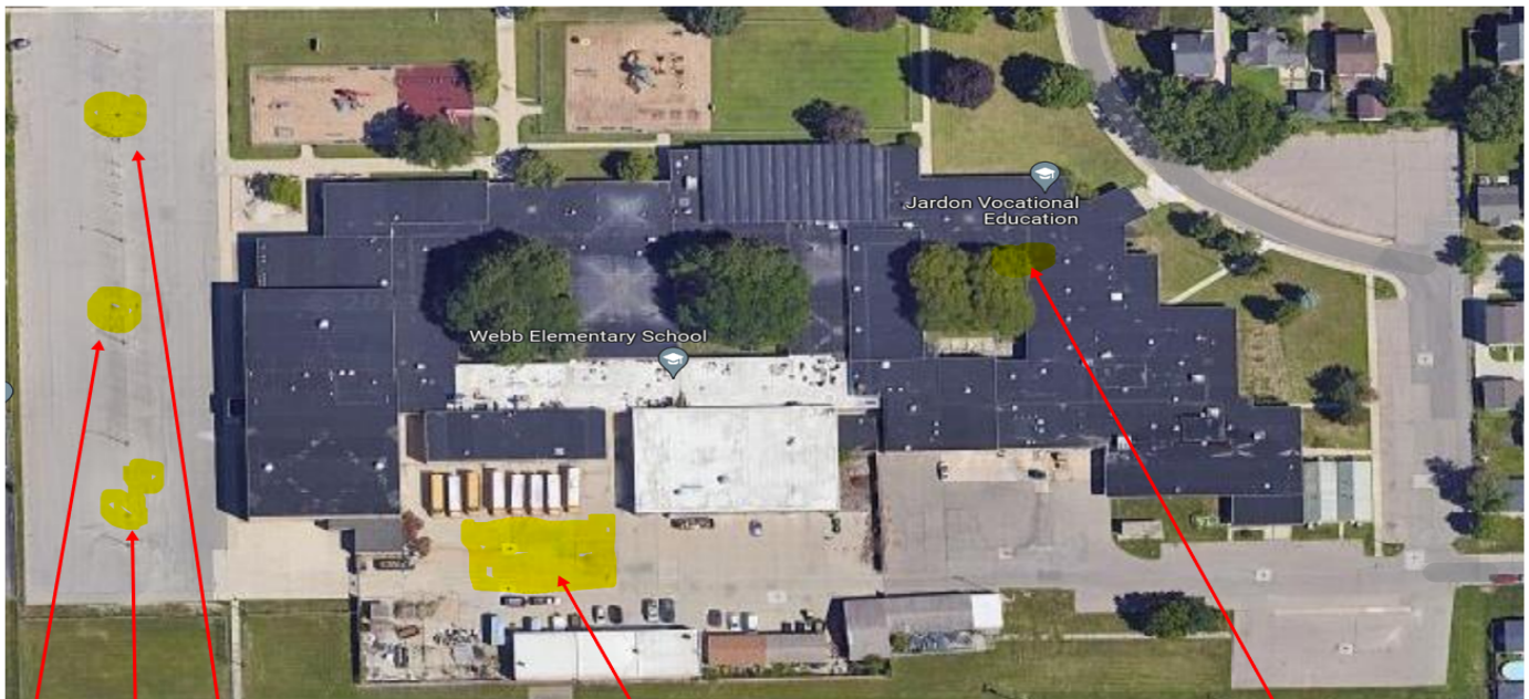
Storm Drain Replacement
