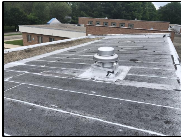
EXISTING ROOFING SYSTEM:
