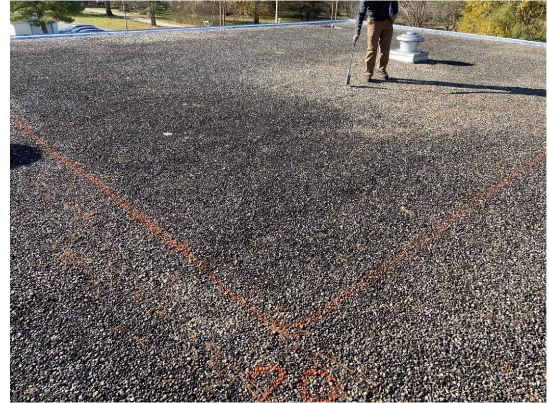
WET AREA IDENTIFIED ON SECTION
