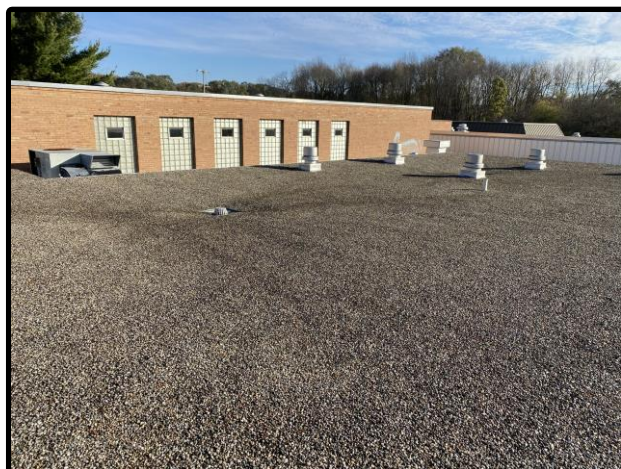
EXISTING ROOFING SYSTEM:
