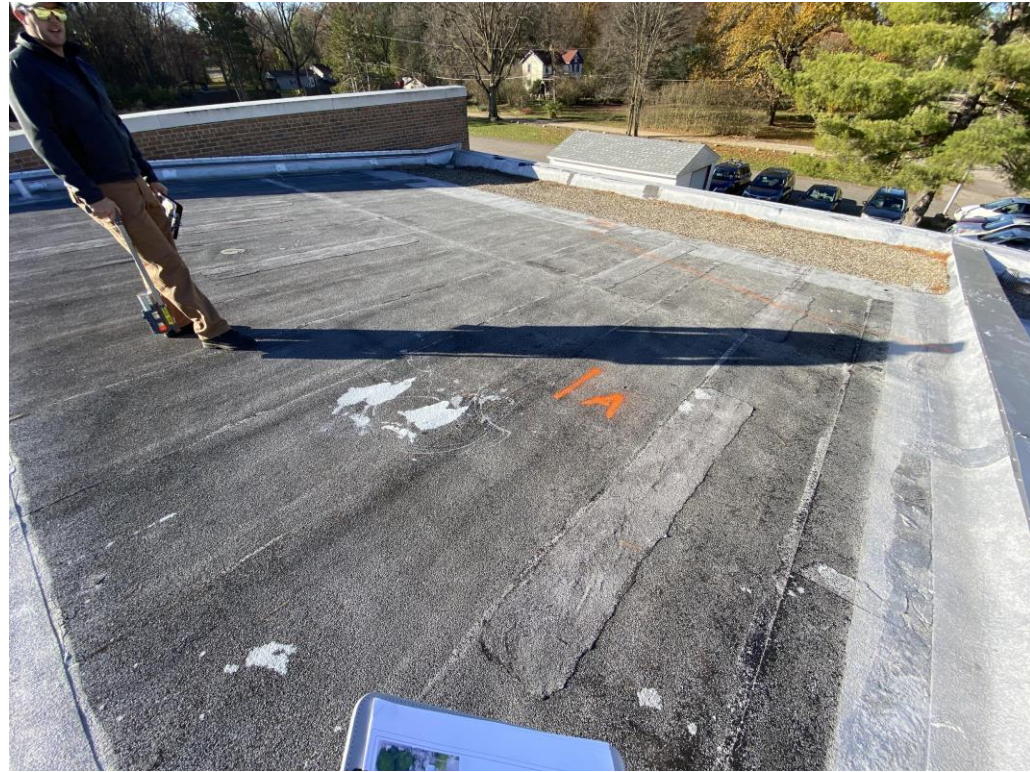
SECTION #1A OVERVIEW. THIS SYSTEM IS A MANCERED MINERAL MOD BIT WITH A FLOOD AND GRAVEL VALLEY
