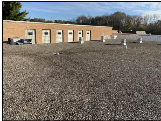
EXISTING ROOFING SYSTEM:
