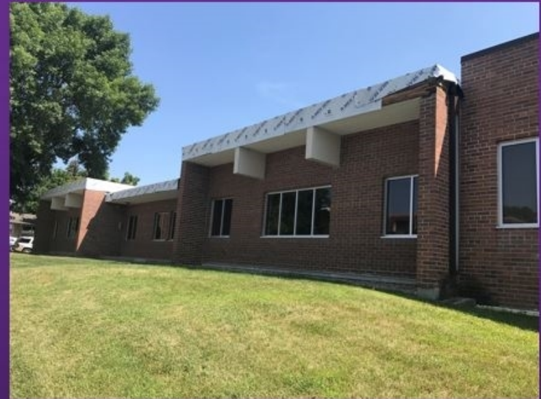
Southview West Wall
