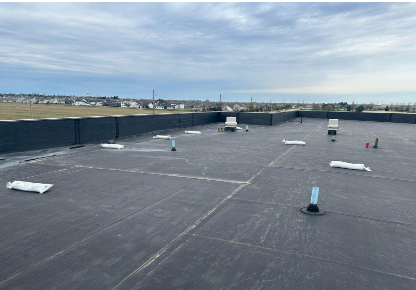
Sandbags holding it in place.
