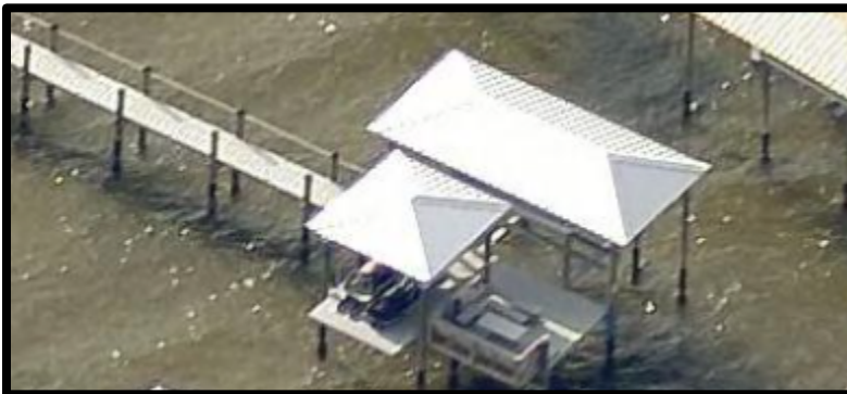
As-Built Dock - Terminal Platform
