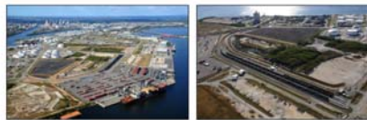
Aerial view of the Tampa Gateway Rail terminal, at the Port of Tampa. The $11 million project was recognized as first-place entry in the development category of the 21st Annual Future of the Region Awards, a program of the Tampa Bay Regional Planning Council, that acknowledges the strongest regional projects in the Tampa Bay area.
