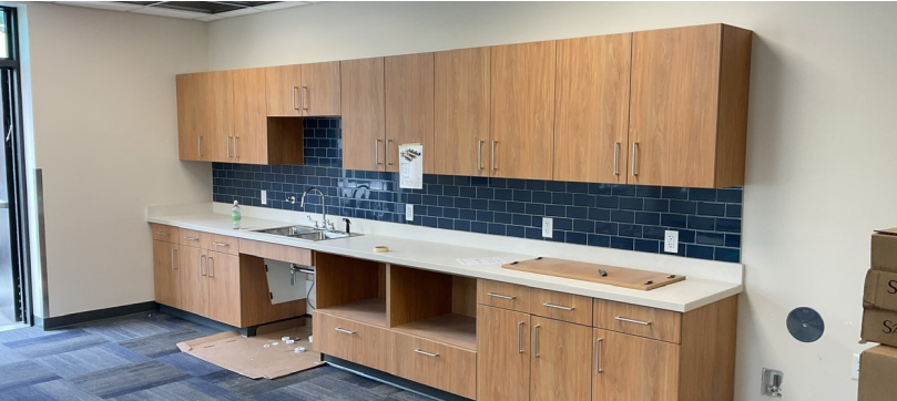
RIVER FALLS TRANSPORTATION CENTER PROGRESS
