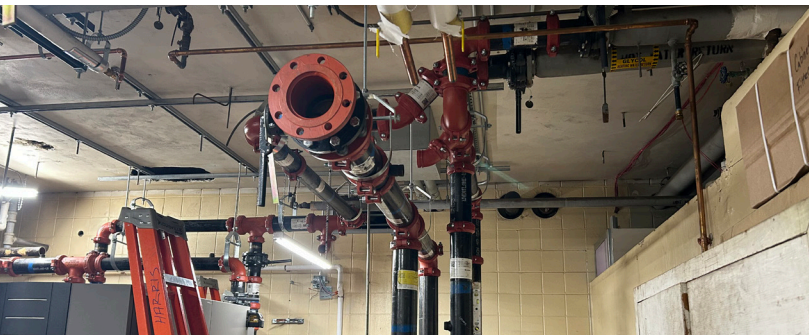
WESTSIDE ELEMENTARY SCHOOL PROGRESS
