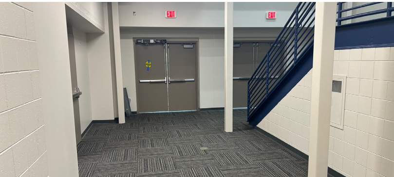
RIVER FALLS HIGH SCHOOL PROGRESS
