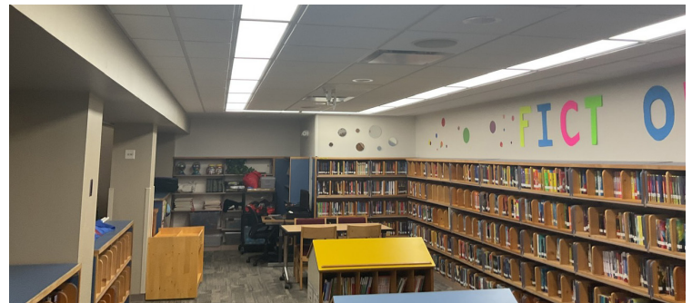
ROCKY BRANCH ELEMENTARY SCHOOL PROGRESS
