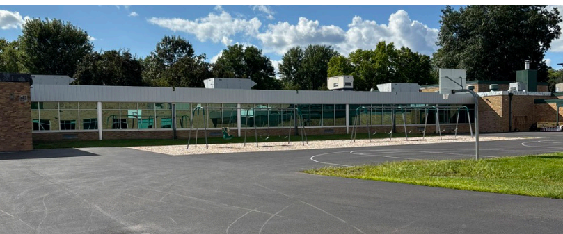
GREENWOOD ELEMENTARY SCHOOL PROGRESS
