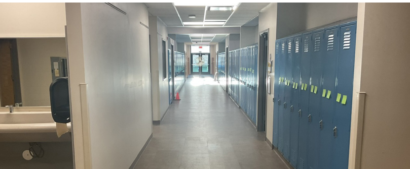
ROCKY BRANCH ELEMENTARY SCHOOL PROGRESS
