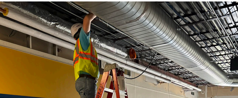
MEYER MIDDLE SCHOOL PROGRESS
