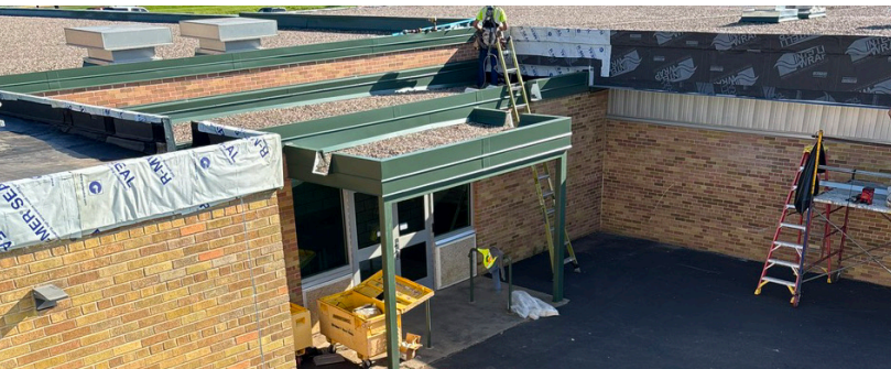
GREENWOOD ELEMENTARY SCHOOL PROGRESS
