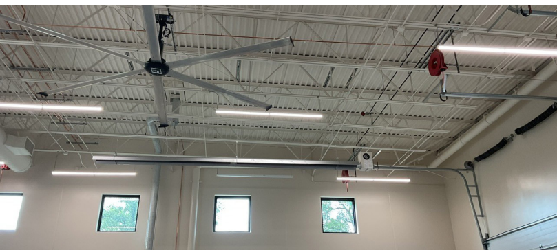
RIVER FALLS TRANSPORTATION CENTER PROGRESS
