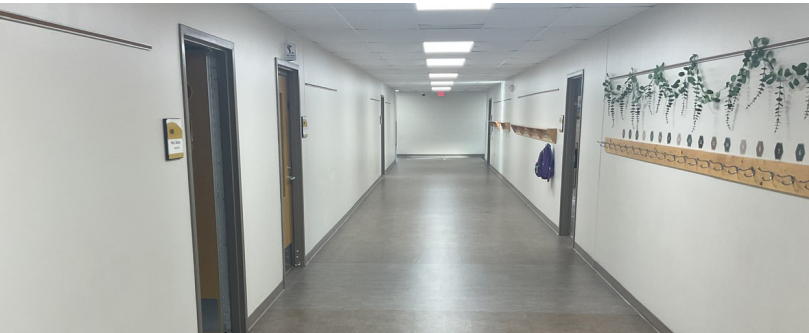
ROCKY BRANCH ELEMENTARY SCHOOL PROGRESS
