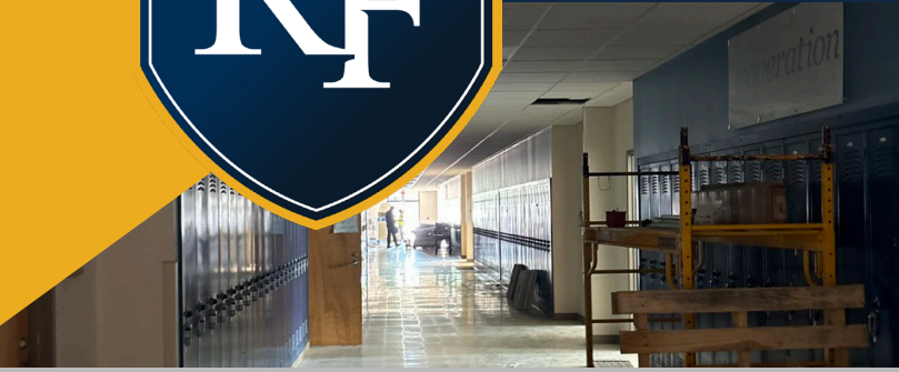
MEYER MIDDLE SCHOOL PROGRESS
