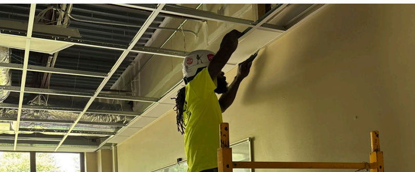
MEYER MIDDLE SCHOOL PROGRESS
