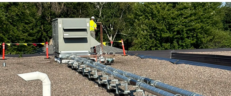
MEYER MIDDLE SCHOOL PROGRESS
