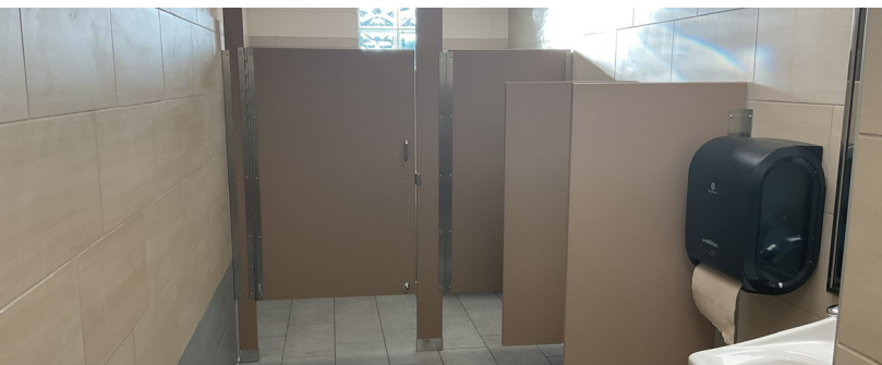
ROCKY BRANCH ELEMENTARY SCHOOL PROGRESS
