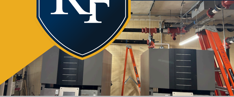
WESTSIDE ELEMENTARY SCHOOL PROGRESS
