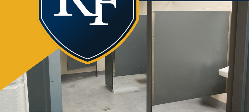
RIVER FALLS TRANSPORTATION CENTER PROGRESS
