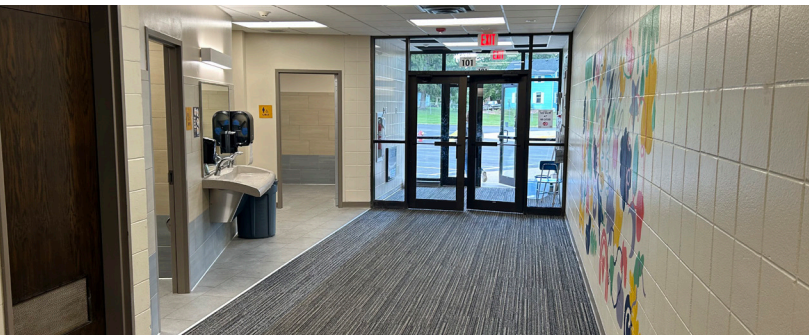
WESTSIDE ELEMENTARY SCHOOL PROGRESS
