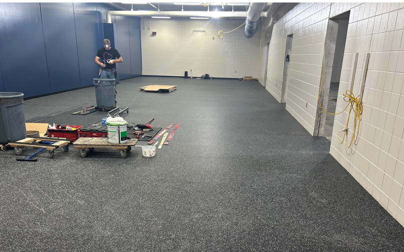
RIVER FALLS HIGH SCHOOL PROGRESS
