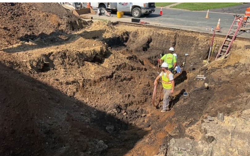
RIVER FALLS TRANSPORTATION CENTER PROGRESS
