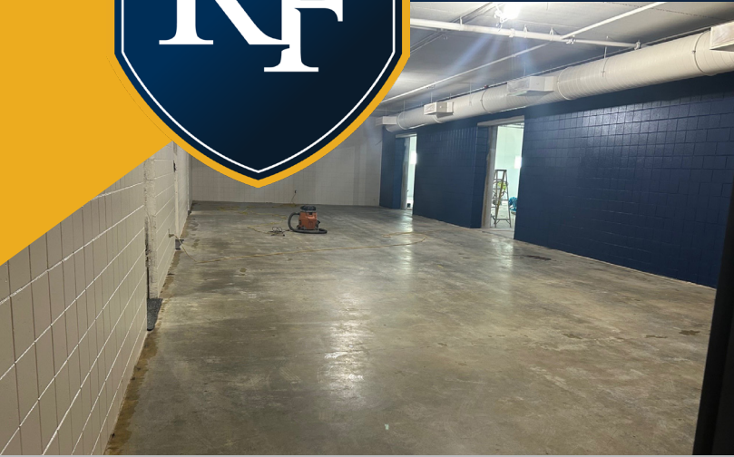
RIVER FALLS HIGH SCHOOL PROGRESS
