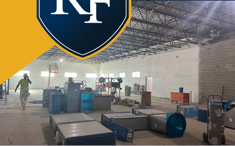
RIVER FALLS HIGH SCHOOL PROGRESS
