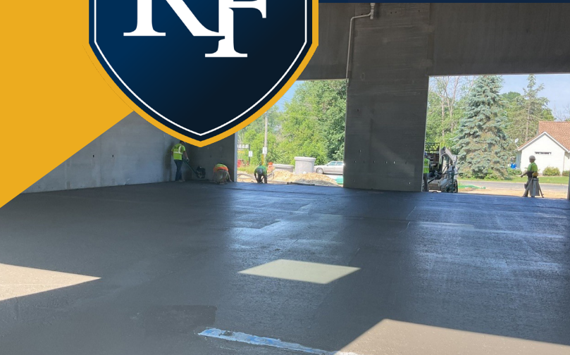
RIVER FALLS TRANSPORTATION CENTER PROGRESS
