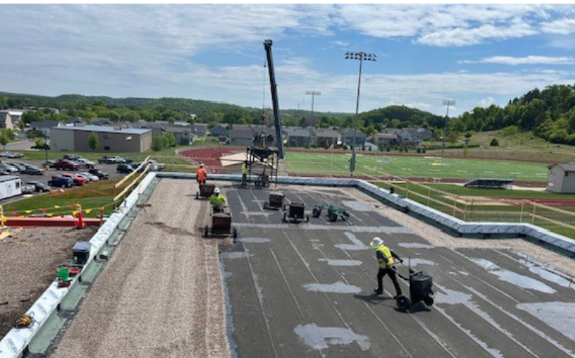
RIVER FALLS HIGH SCHOOL PROGRESS
