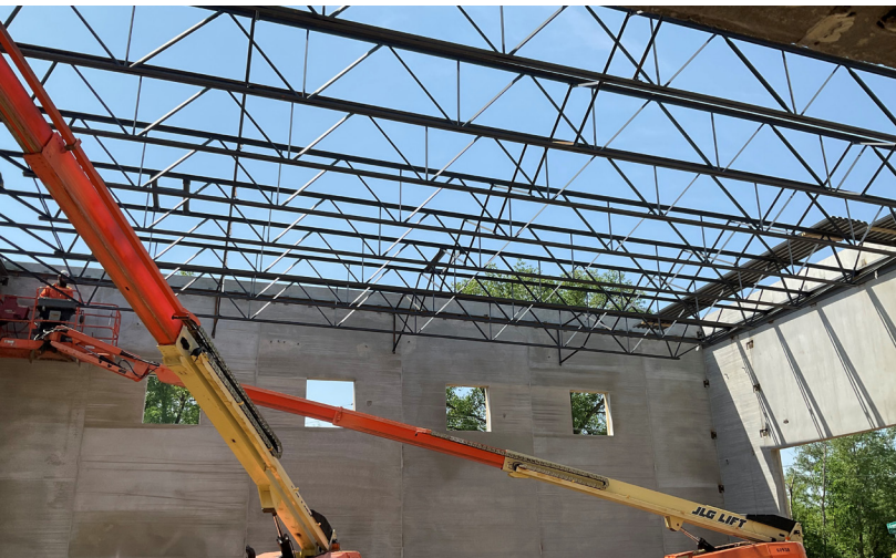
RIVER FALLS TRANSPORTATION CENTER PROGRESS
