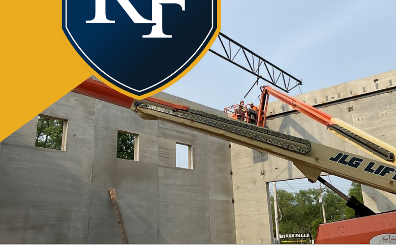
RIVER FALLS TRANSPORTATION CENTER PROGRESS
