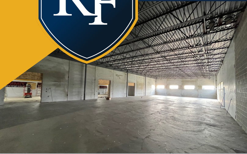
RIVER FALLS HIGH SCHOOL PROGRESS
