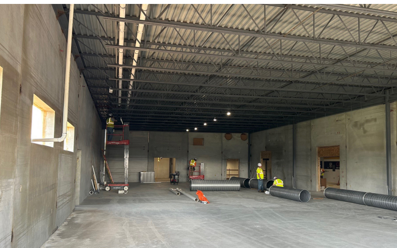
RIVER FALLS HIGH SCHOOL PROGRESS
