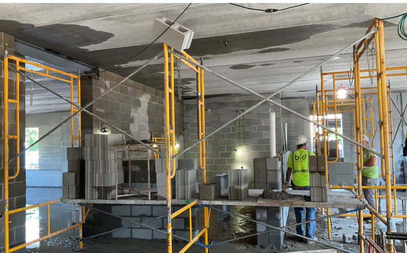
RIVER FALLS TRANSPORTATION CENTER PROGRESS
