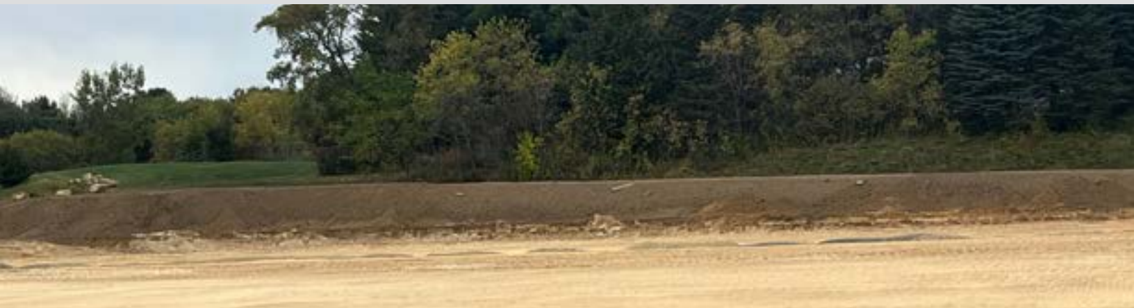
DEMOLITION OF THE TENNIS COURTS
