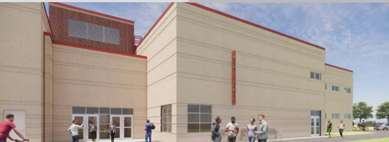
RIVER FALLS HIGH SCHOOL MULTIPURPOSE ROOM - ENTRANCE
