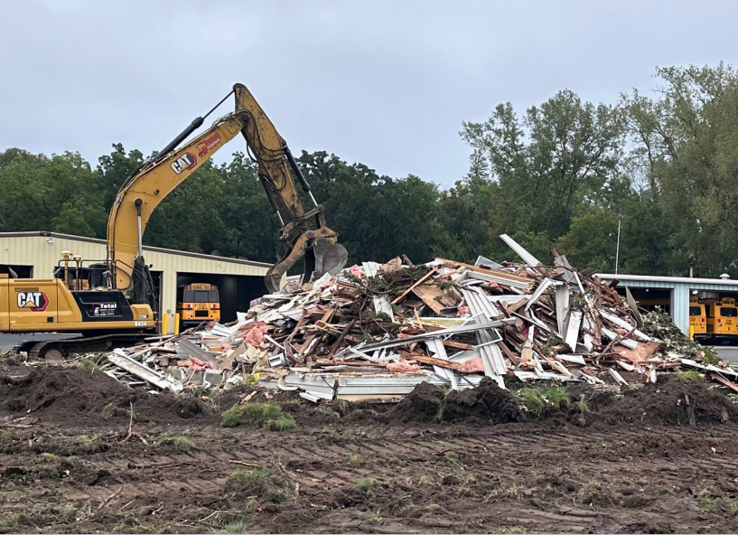
DEMOLITION AT NEW TRANSPORTATION CENTER SITE
