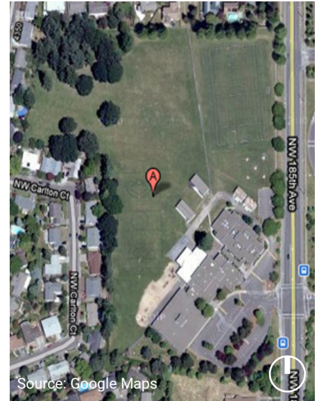
IMAGE: Rock Creek Elementary School
