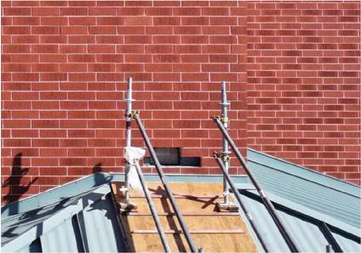
OPENING #7: Standing Seam Roof Ridge
