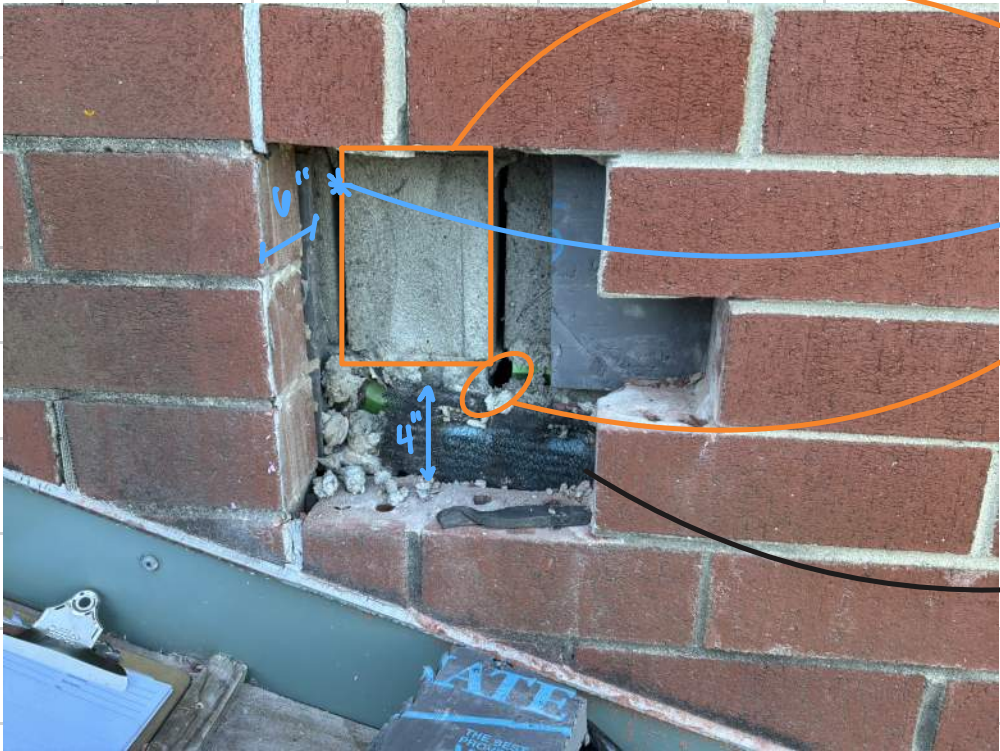
Opening #3 west entrance bottom of skylight
