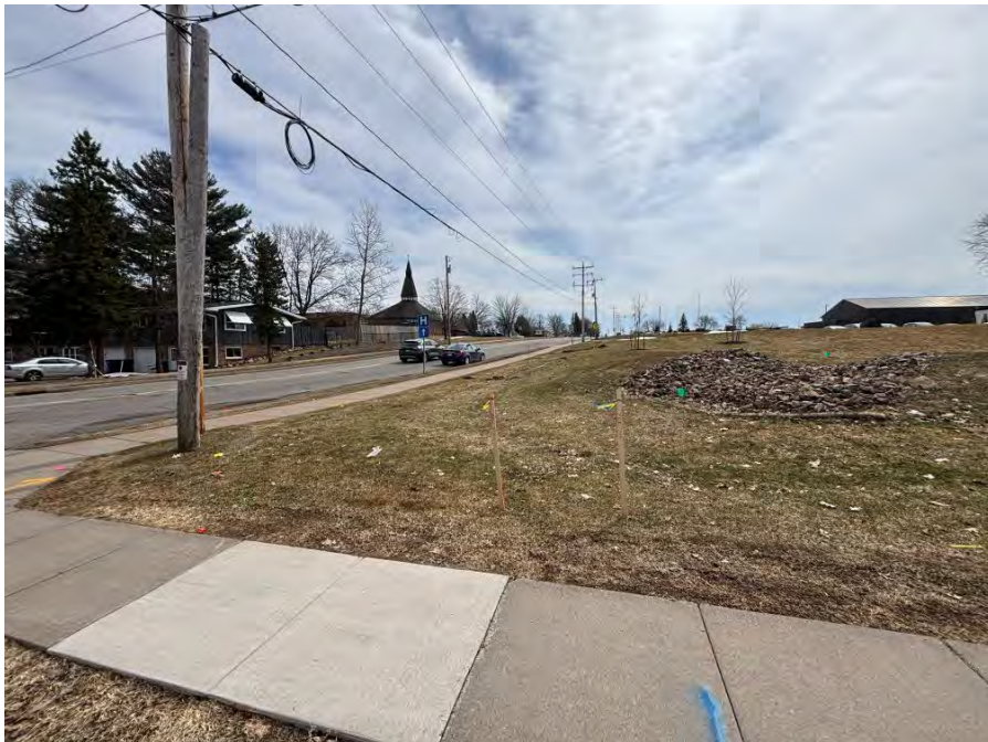
The TLE and fee acquisition area at the corner of Jelinek Ave and Alderson St. Alderson St can be seen in the background.
