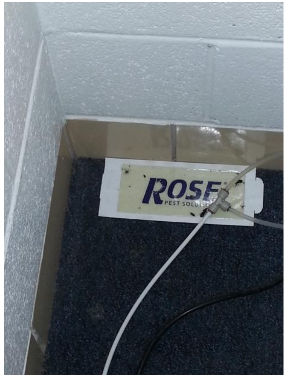
Photo 16 – Lounge: Roach trap in south corner
