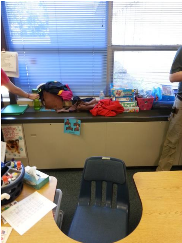
Photo 15 – Room 120 Obstructed uni-vent
