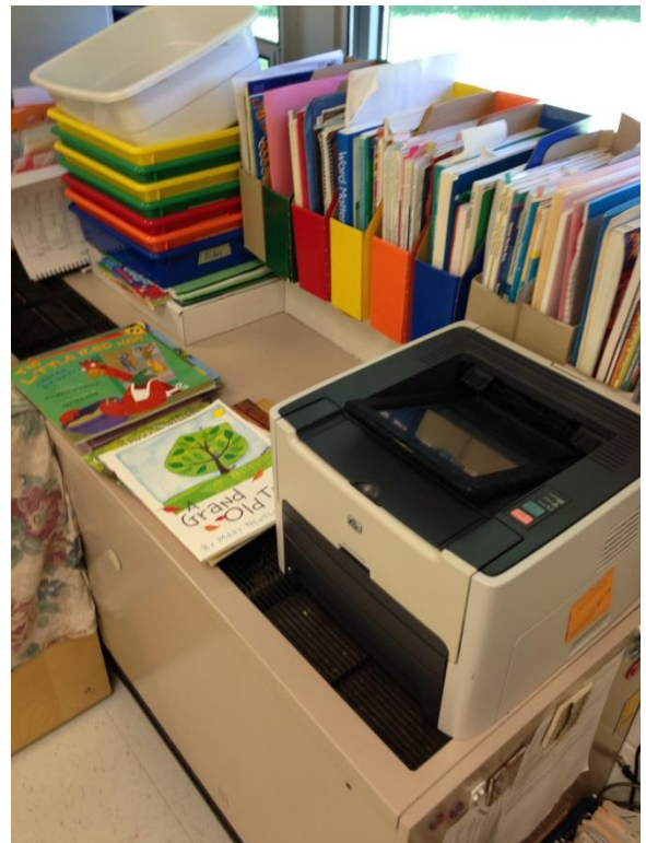
Photo 60 – Room 139 - Obstructed uni-vent
