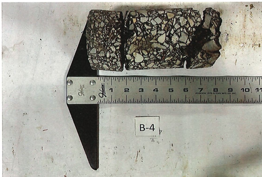
Pavement Core B-4: Spaulding Elementary School
