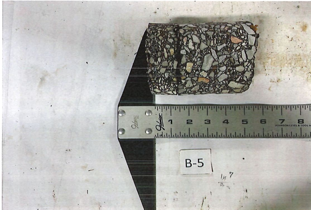
Pavement Core B-5: Spaulding Elementary School
