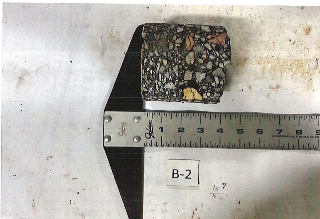
Pavement Core B-2: Spaulding Elementary School
