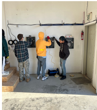
Students learning how to wire electrical panales
