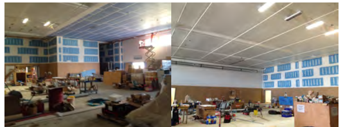
Interior shots of the old and new parts of the gym.
