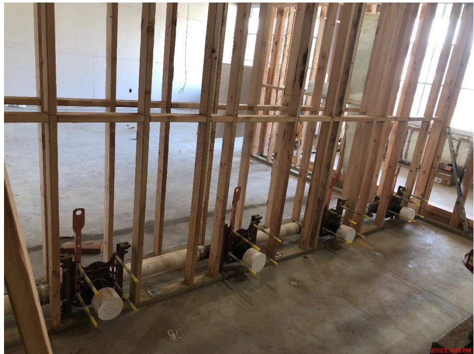
CHHS – Bathroom fixture mounts in wall
