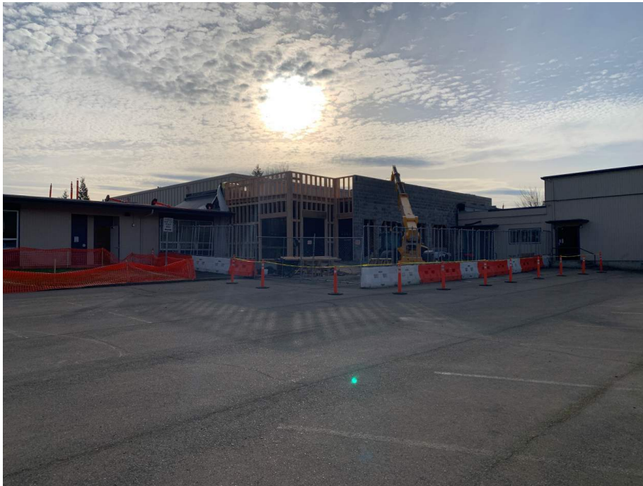
New Administration Wing – View from area of new visitor parking
