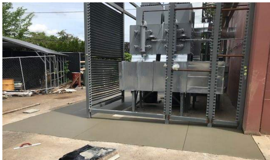
New slab at dust collector screen wall
