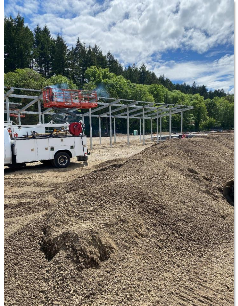
Bike Shelter Steel Erection
