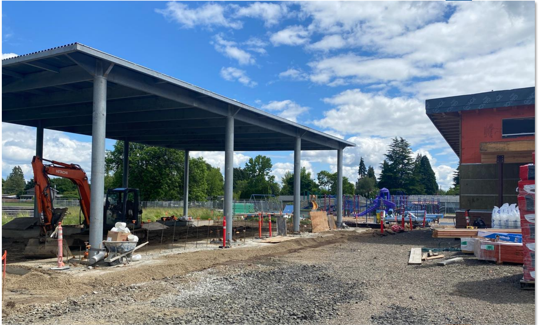
Play Structure and End of the New Addition
