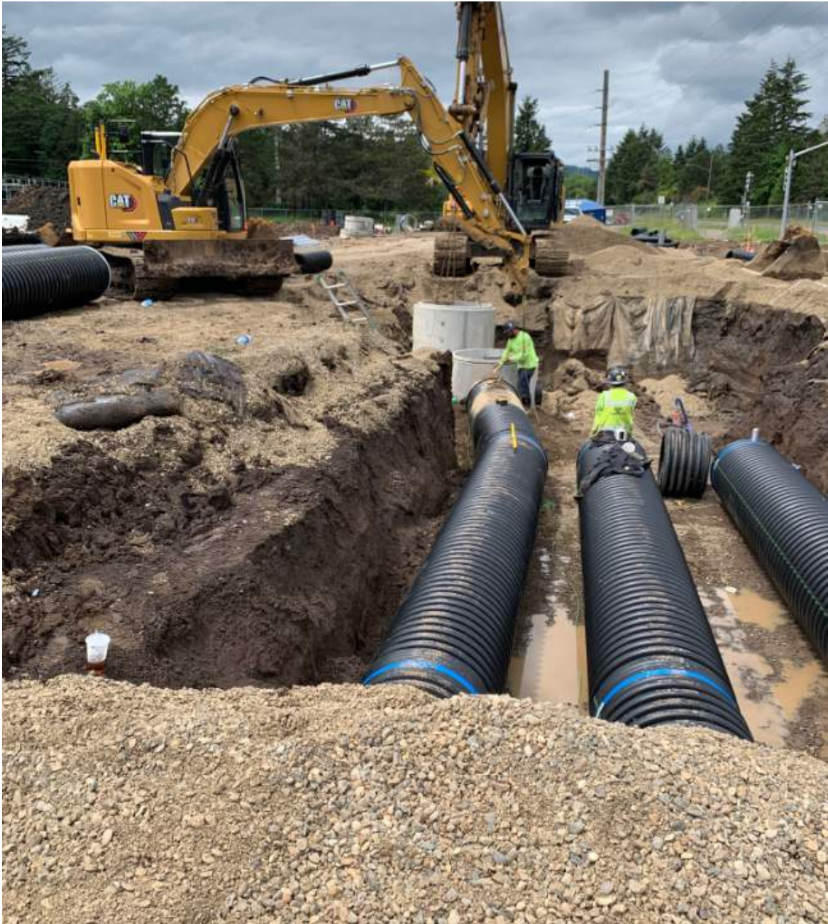
Storm Detention Facility
