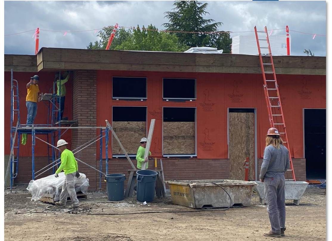
Last of the Masonry at the New Addition
