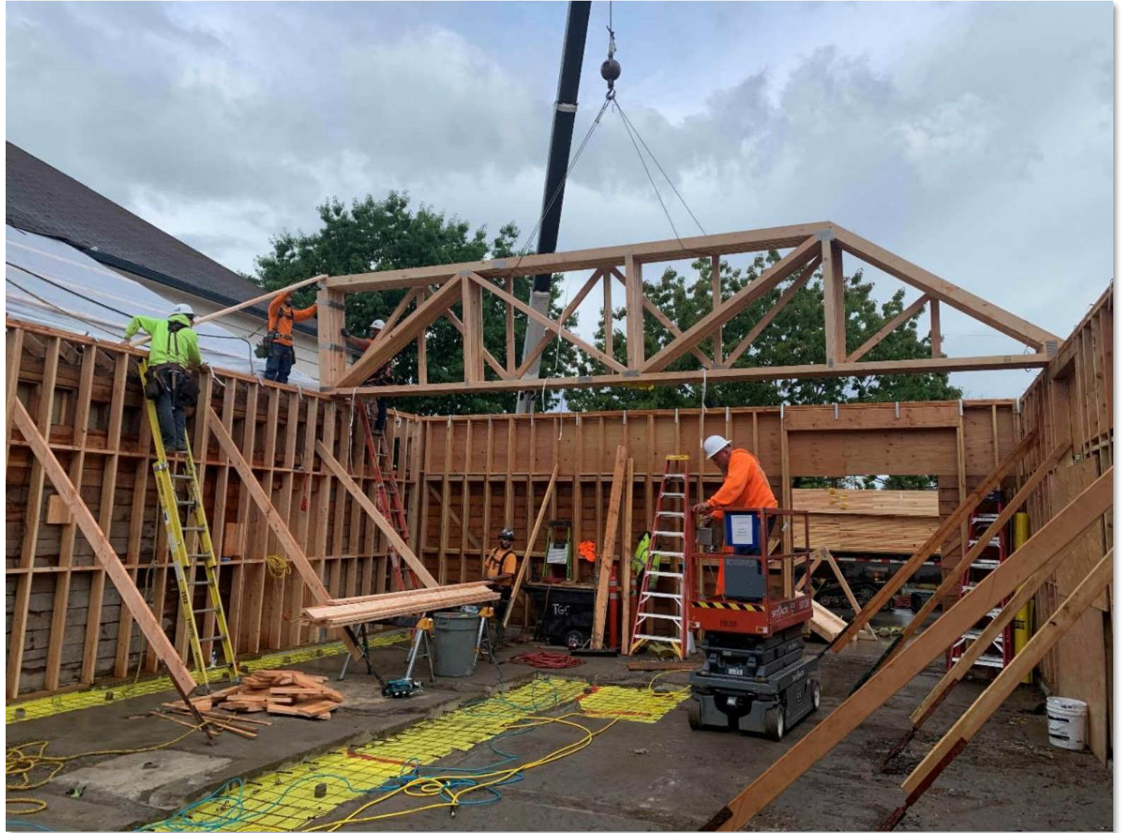
Science Classroom Trusses Flying Into Place
