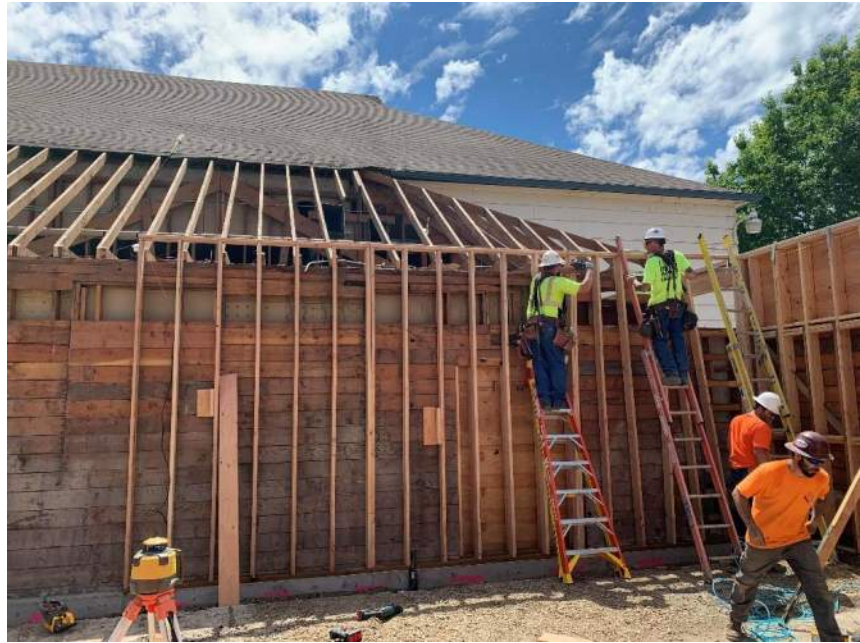
New framing at hallway near science room
