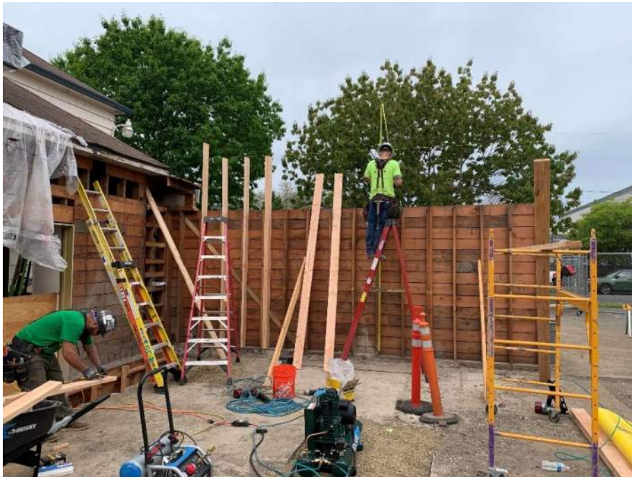
Extending science room exterior walls
