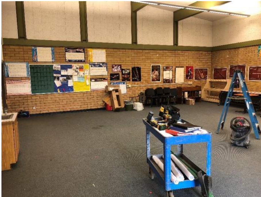
Band Room Cleared for early construction start
