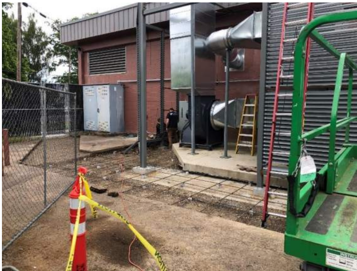
Prepped for new slab at dust collector screen wall
