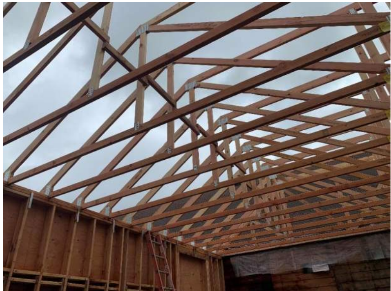
New science room trusses
