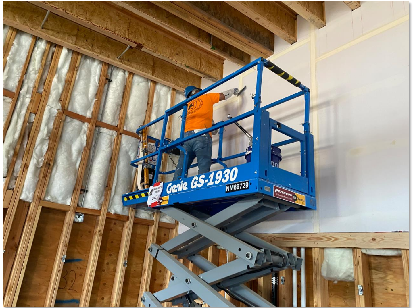
Classroom Sheetrock Mudding
