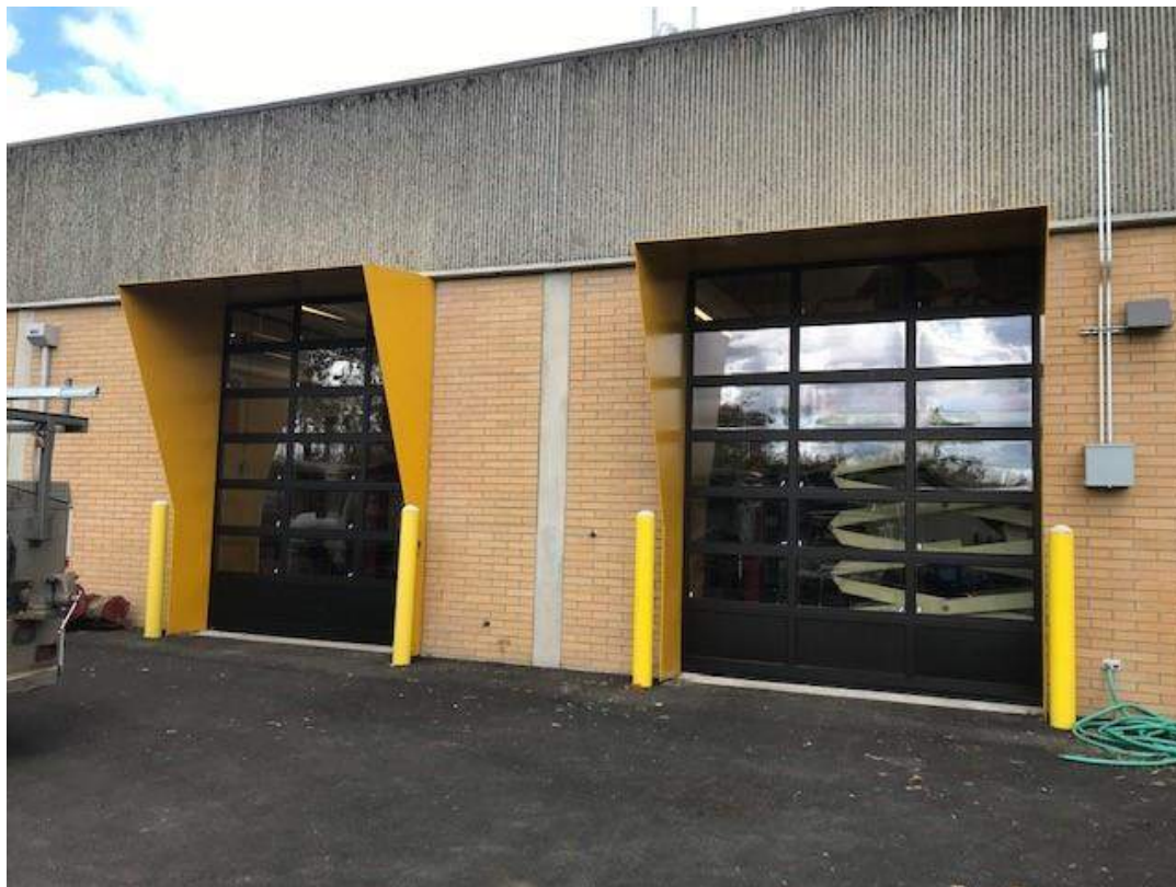
Autos Overhead Doors Installed
