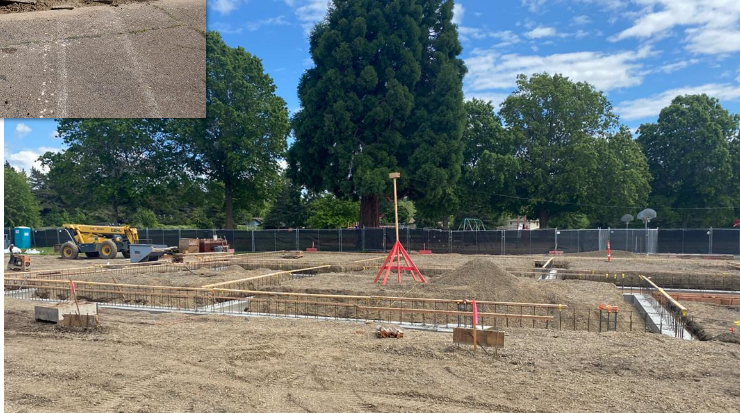
Concrete Footings Poured at New Addition
