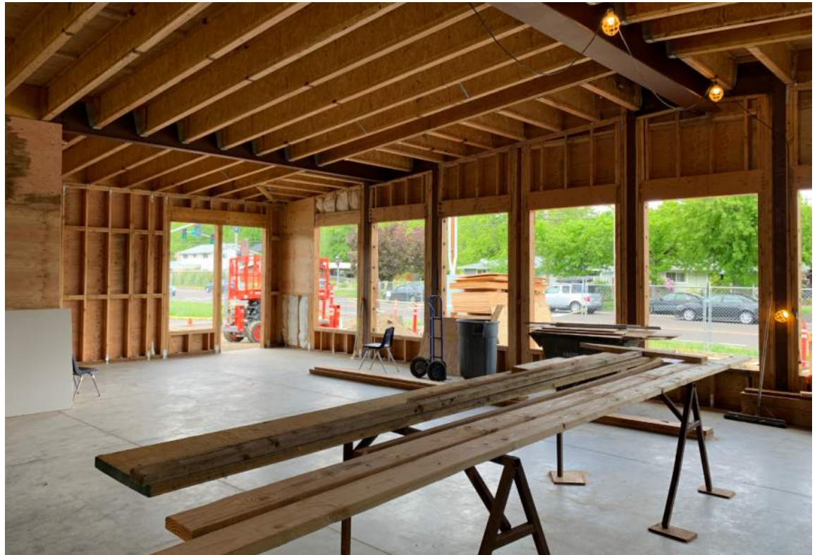
A cafeteria with lots of daylight!
