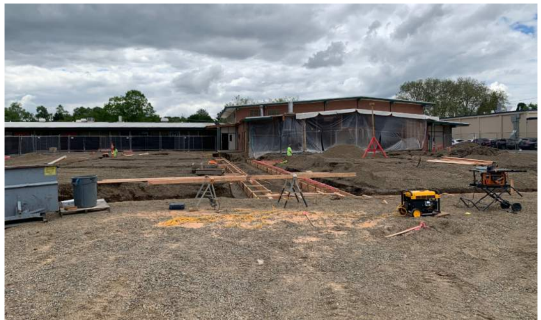
Locker Room Demo & Footing Prep
