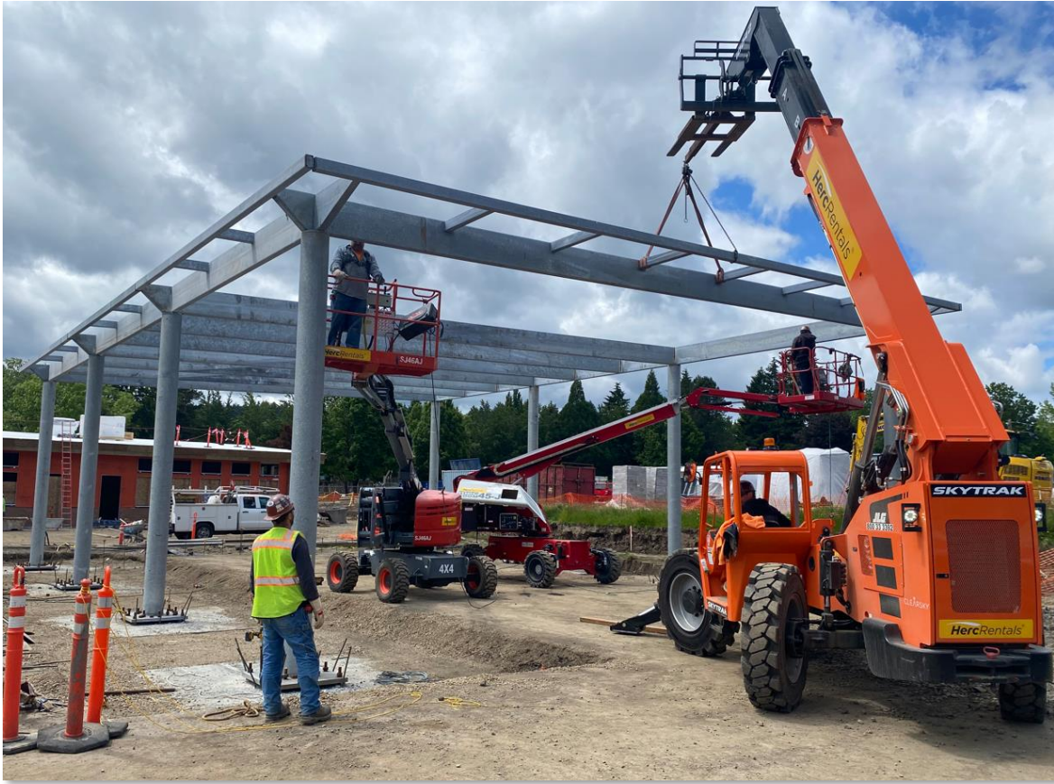
Play Structure Steel Erection
