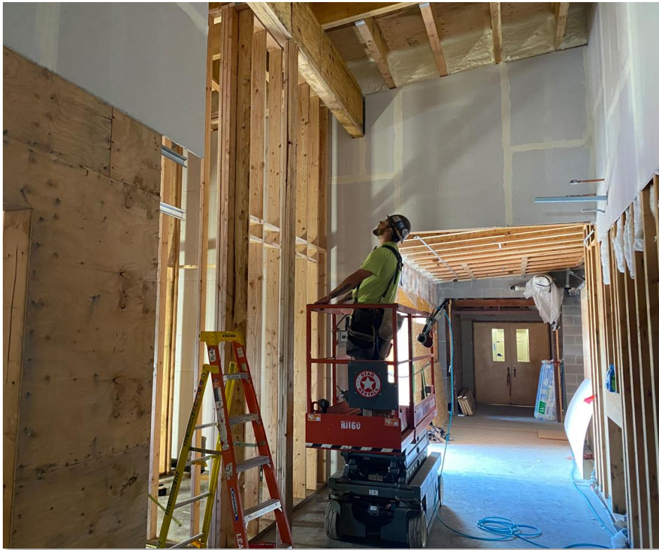
Corridor Rough-in Work
