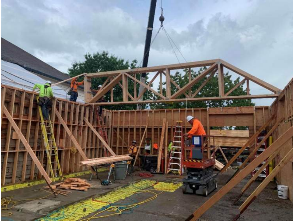
New science room – setting trusses
