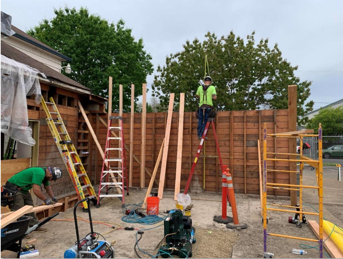
Framing Begins on New Science Room
