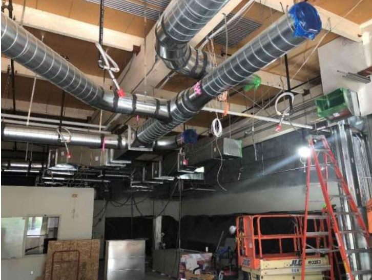
CVHS – new HVAC in ceramics ceiling
