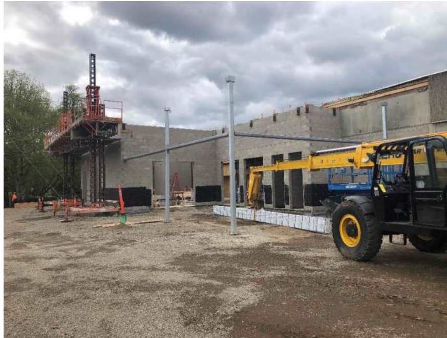
CVHS – New addition and covered work area
