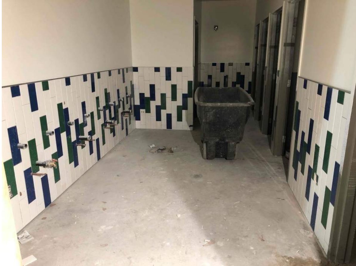
Garfield – Area C new restroom progress
