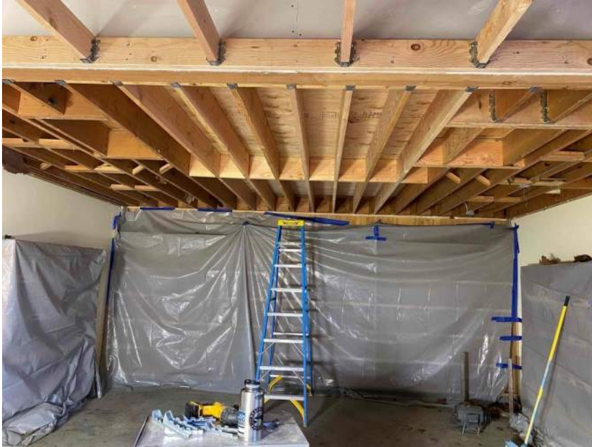
New HVAC mezzanine infill framing
