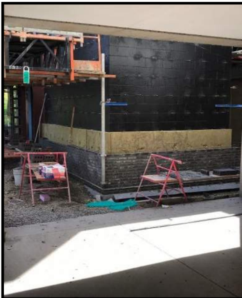
CVHS – (left) brick installing at elevator and (right) walkway framing to 2 nd level
