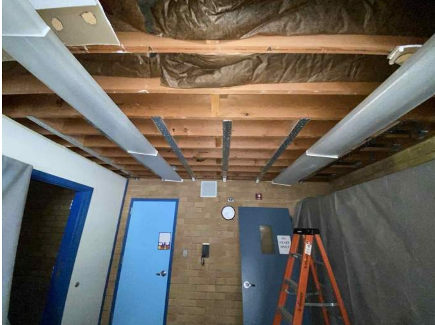
CMS seismic work installing in ancillary rooms on N & S ends of Library
