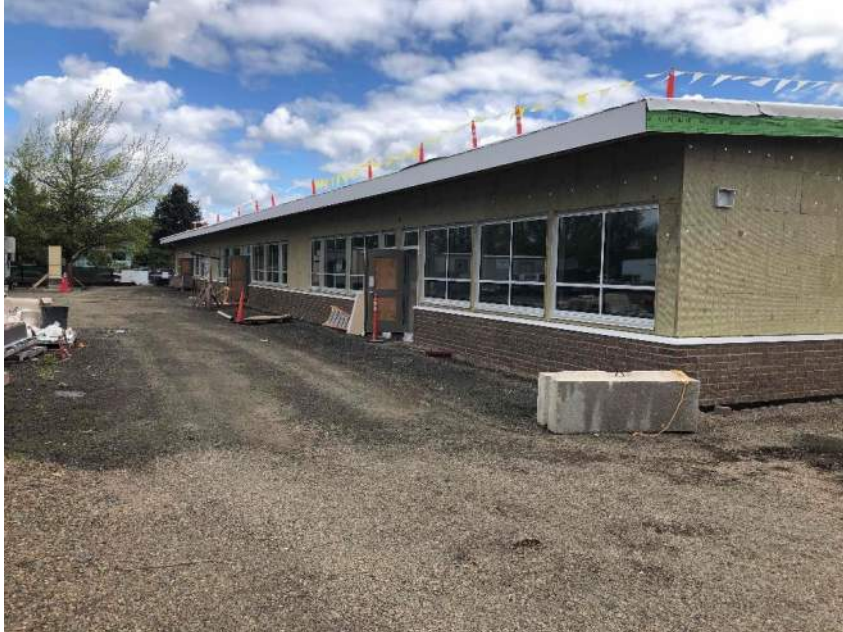
Garfield Area C – exterior glass installation- ready for siding
