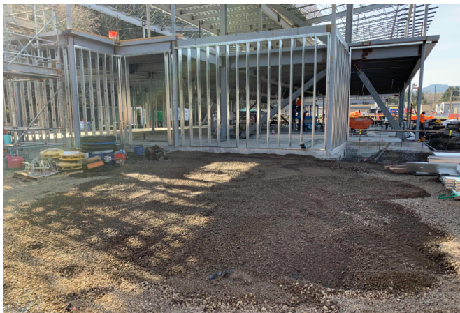
Start of wall construction
