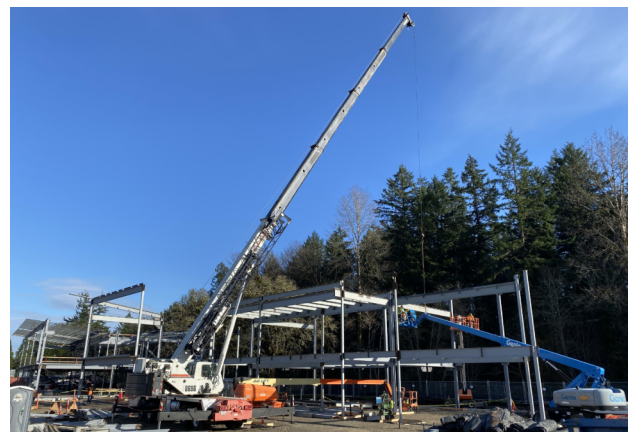
Steel Erection at Husky
