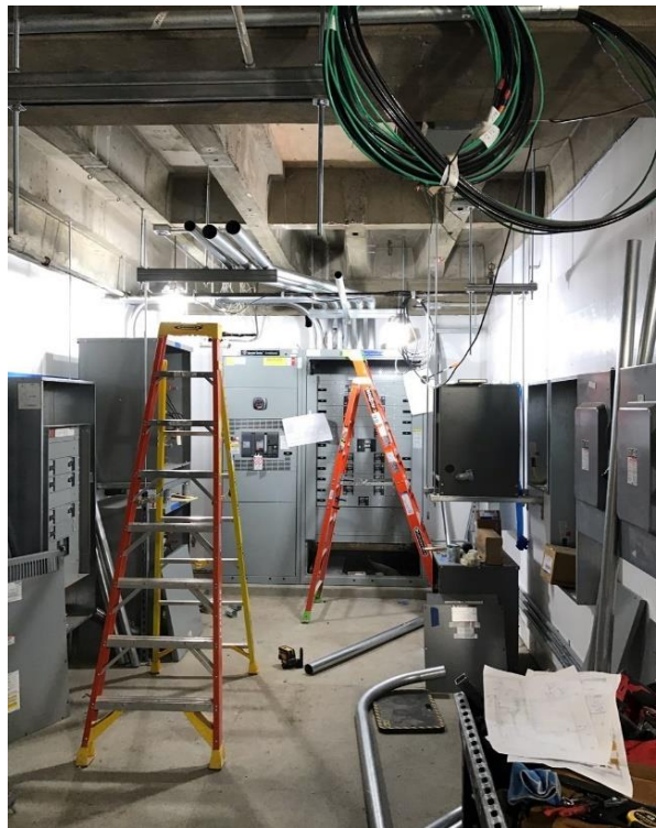
CVHS – Electrical room taking shape
