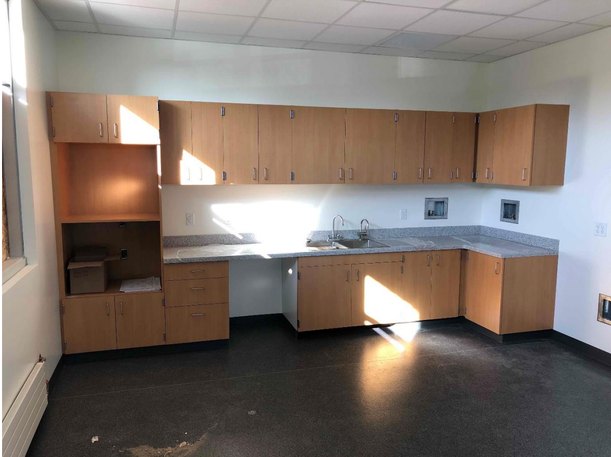
Staff break room casework installed
