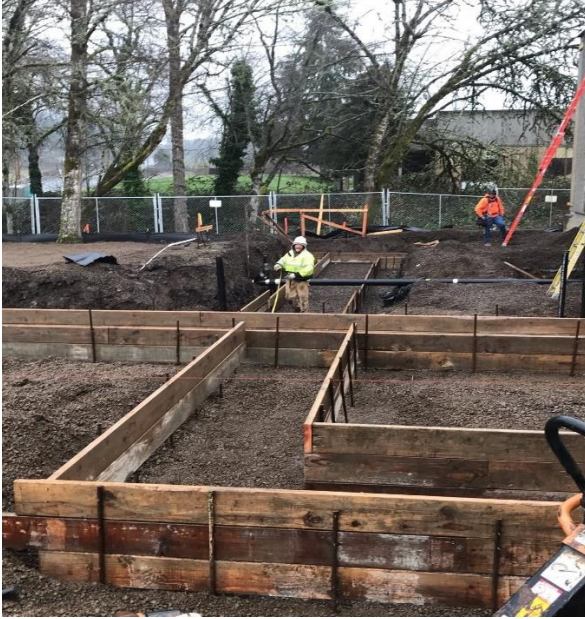
CVHS Outdoor work area – footings to be placed soon
