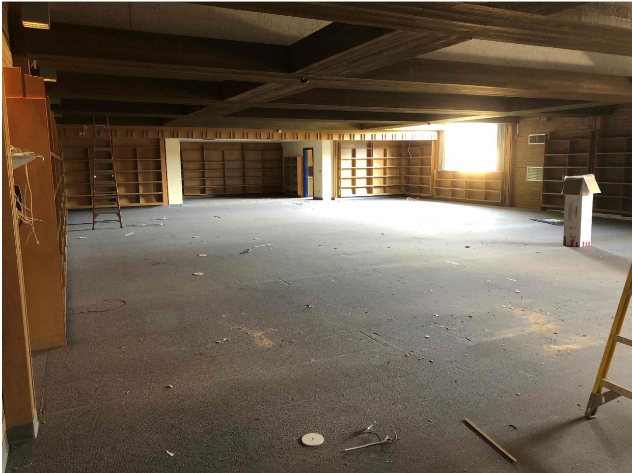
Library cleared for new construction
