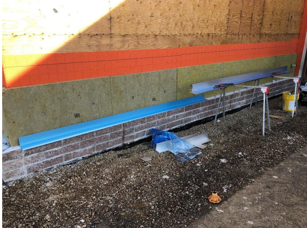
Garfield New Addition - exterior skin - early installation
