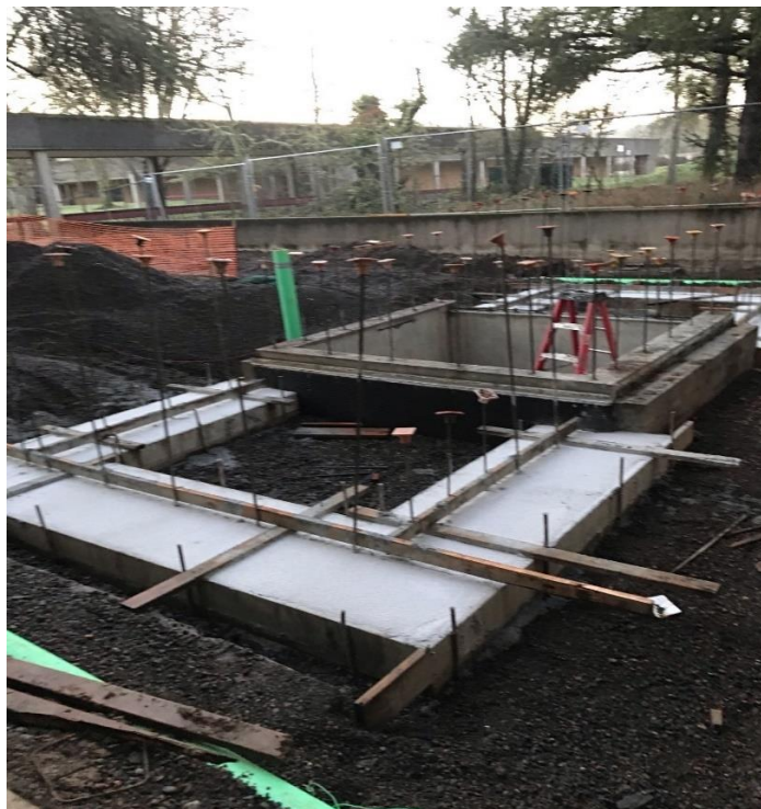
CVHS Building A -Elevator area taking shape
