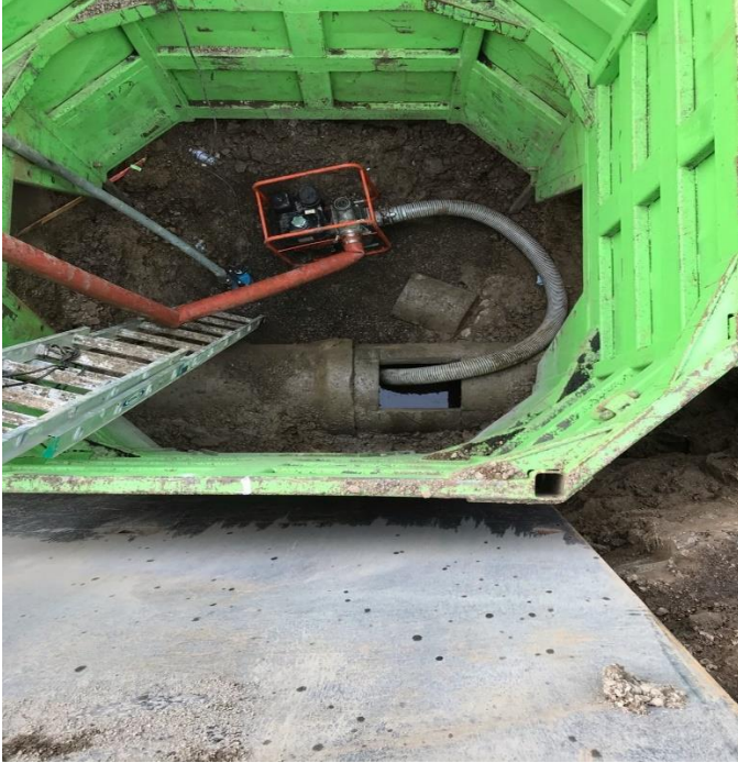
CVHS Exterior Storm Drain tie in- It is DEEP
