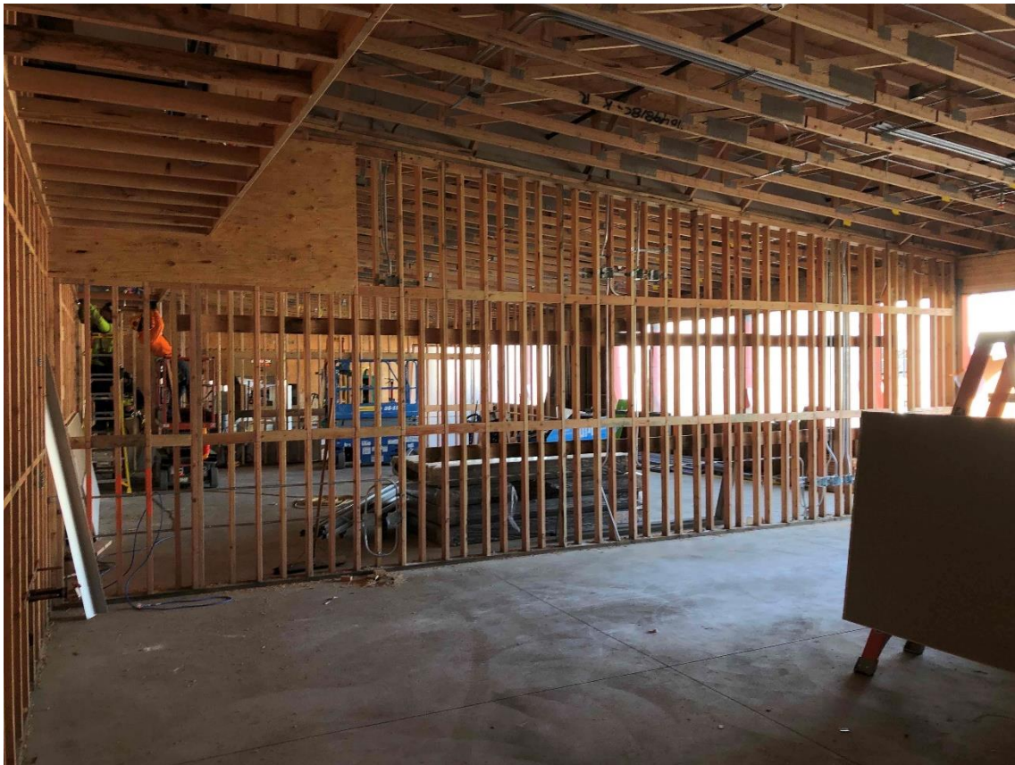
Area C North side interior framing – plywood on many walls already
