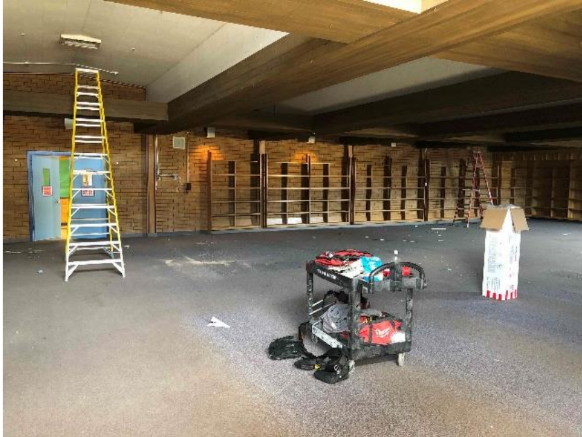
Lighting removed from Library to make way for new
