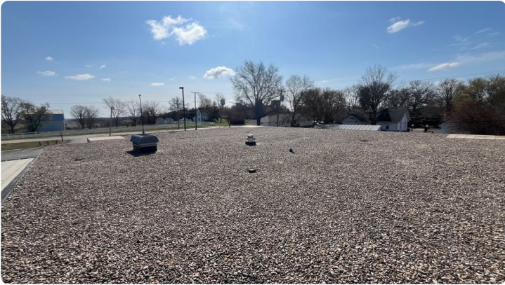
Photo showing overview of Area 03 roof.
