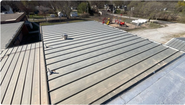
Photo showing overview of Area 11 roof.
