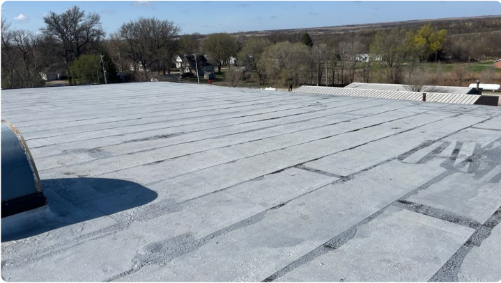
Photo showing overview of Area 10 roof.
