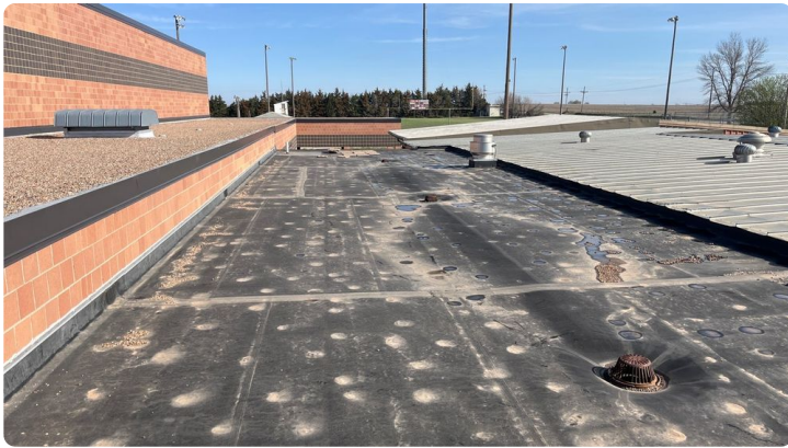
Photo showing overview of Area 05.
