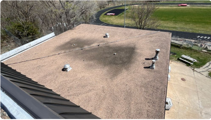
Photo showing overview of Area 03 roof.
