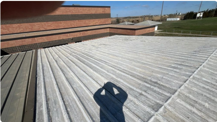
Photo showing additional overview of Area 04 roof.
