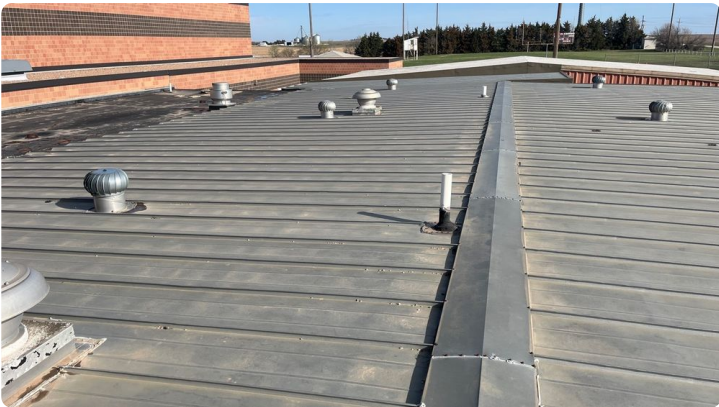
Photo showing additional overview of Area 02 roof.
