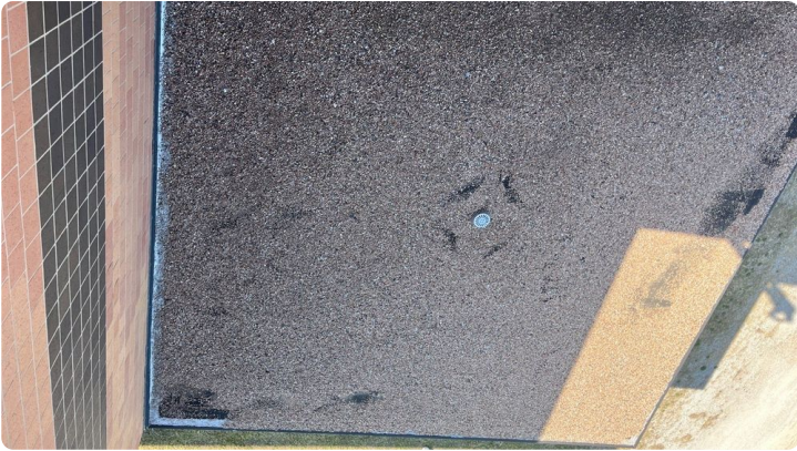
Photo showing overview of Area 08 roof.
