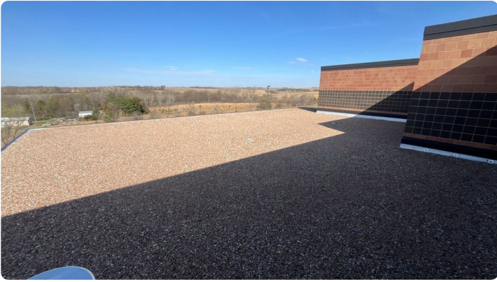
Photo showing overview of Area 09 roof.
