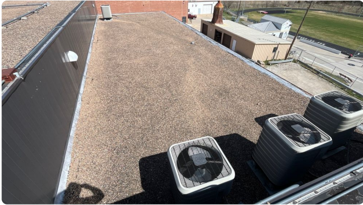
Photo showing overview of Area 05 roof.
