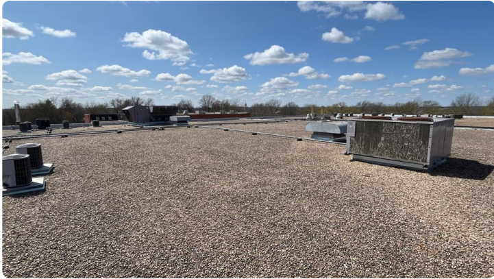
Photo showing overview of Area 01 roof.
