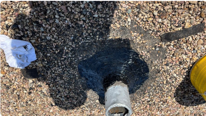
Photo showing repair made to the soil stack.
