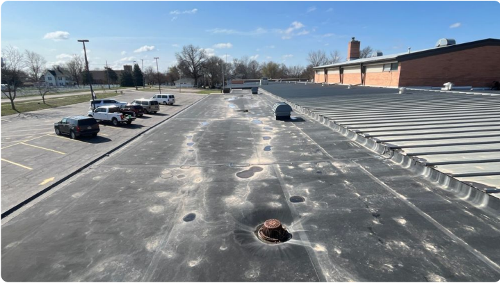
Photo showing overview of Area 01 roof.
