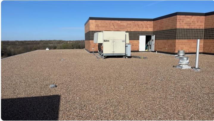
Photo showing overview of Area 06 roof.
