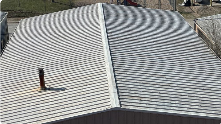
Photo showing overview of the middle roof.
