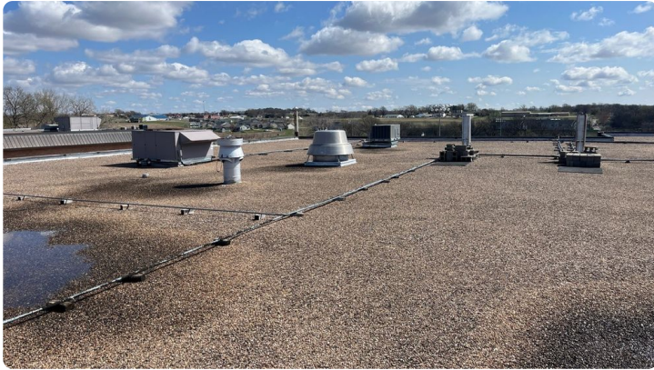
Photo showing overview of Area 04 roof.
