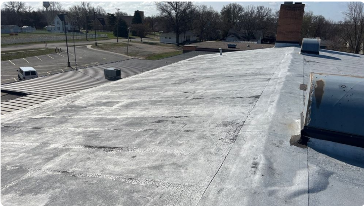
Photo showing additional overview of Area 10 roof.
