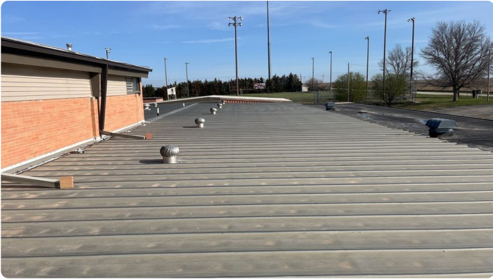
Photo showing overview of Area 02 roof.
