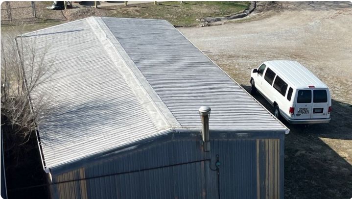
Photo showing overview of the West roof.
