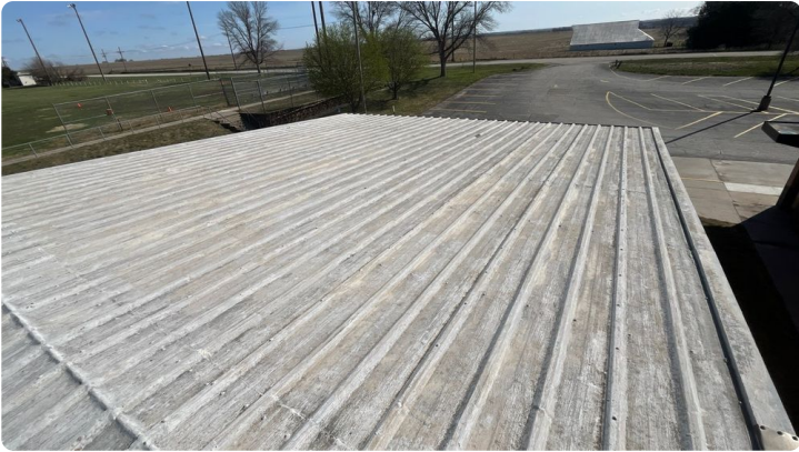
Photo showing overview of Area 04 roof.
