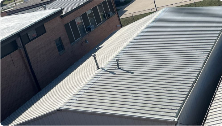
Photo showing overview of the East roof.
