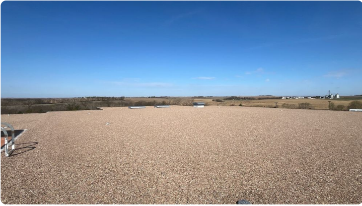
Photo showing overview of Area 07 roof.
