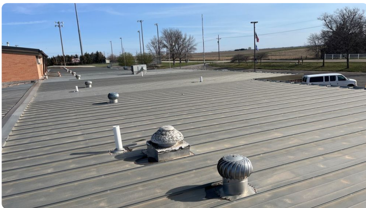
Photo showing additional overview of Area 02 roof.
