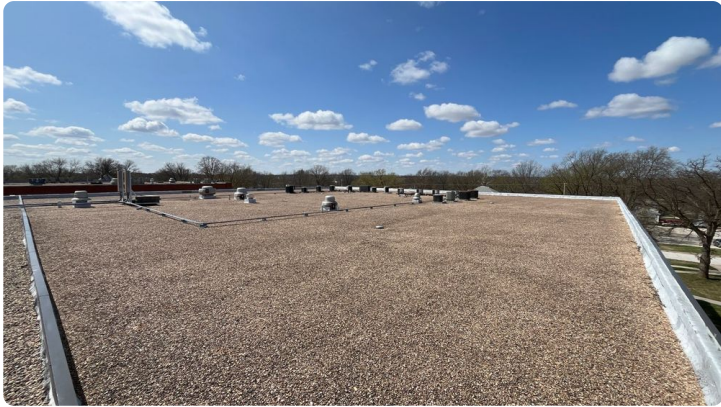
Photo showing overview of Area 02 roof.
