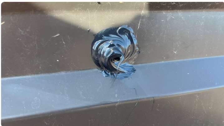
Photo showing the hole in the metal counter flashings repaired.
