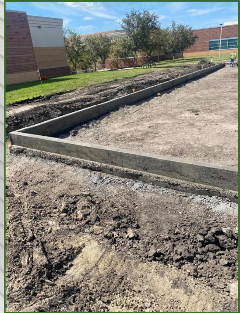
New Curbing installed for relocated playground
