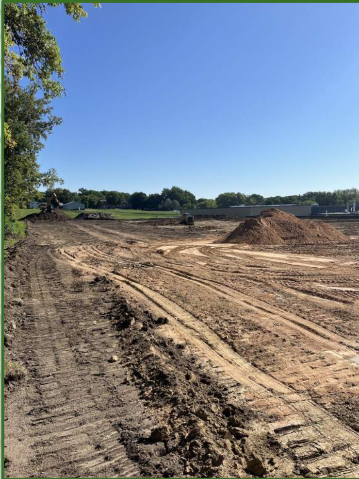
Initial removals of topsoil and aggregate lime for MS bus loop
