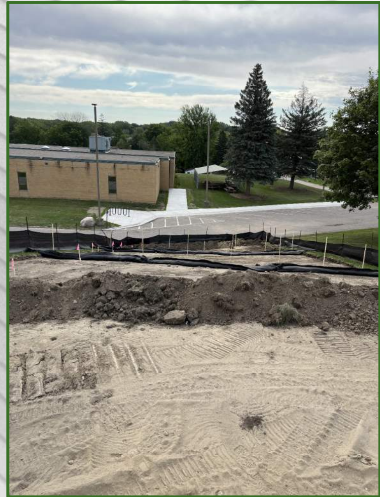
Topsoil removed and erosion control installed in preparation of new sidewalk
