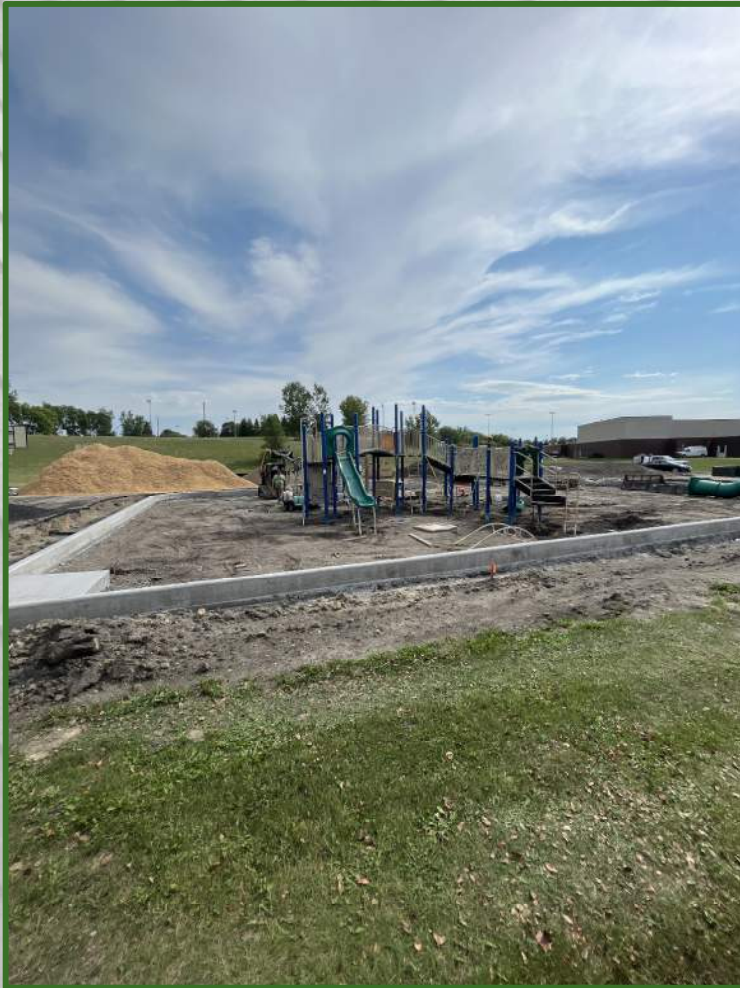
Playground reinstatement underway
