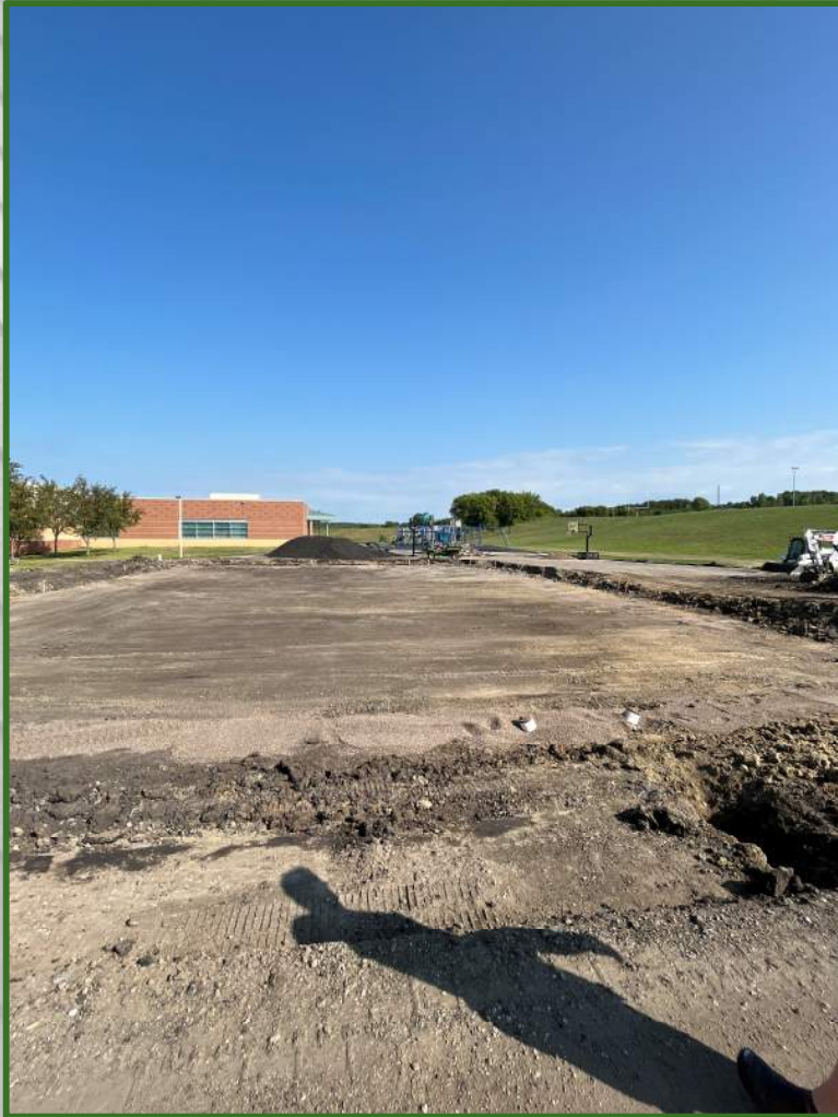
Removal of topsoil and drain tile installed for relocated playground
