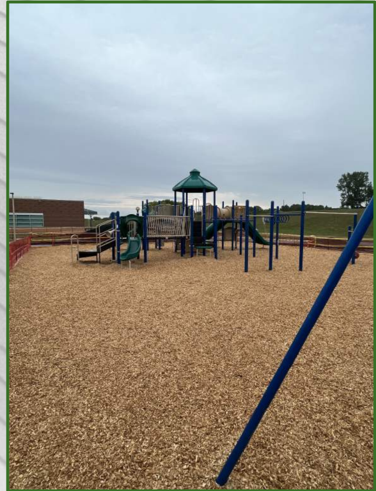
Reinstatement complete with mulch surfacing and fencing installed
