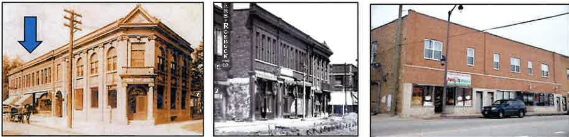
Left: Looking west at 501 Lake Street, Maywood State Bank (right) and 505 (arrow) Lake Street. Middle: Looking east at 505 Lake Street. Right: 505 Lake Street in 2024. Historic images from Maywood Public Library Archives
