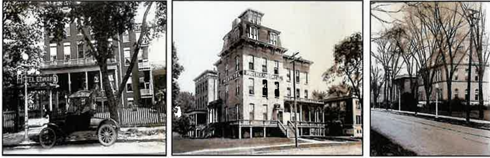
Left: is Hotel Edward that faced St. Charles Road, east of 5 th Avenue. Middle: is the former Maywood Hotel after the conversion to the Phoenix Hospital. Hotel Edward is to the left of the building. Right: is the Maywood Public Library (1905) on the left and the Village Hall (1897) on the right. Images from Maywood Public Library Archives.
