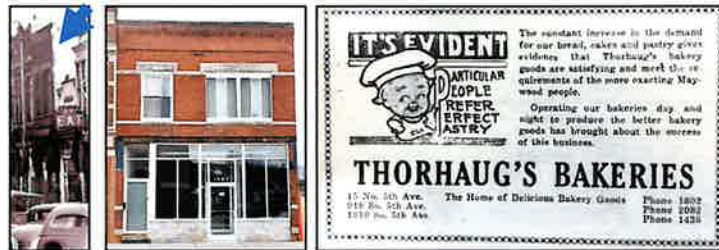
Left: Thorhaug Building at 15 North 5 th Avenue. Image from Maywood Public Library Archives. Middle: Thorhaug Building in 2024. Right: Ad for Thorhaug’s Bakeries. From Maywood Herald.
