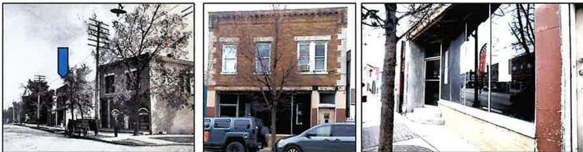
Left: Froemming Building (arrow) and original building in vacant lot at 516 Lake Street from 1909. Image from Maywood Public Library Archive. Middle: Froemming Building in 2024. Right: Close up of late 1920s storefront remodeling in 2024.
