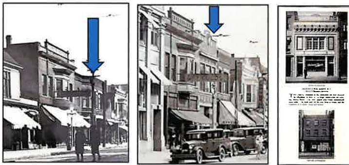
Left: Gustavison Building at 17 North 5 th Avenue prior to 1925. Middle: Gustavison Building after 1925. Right: Ad from Architectural Terra Cotta Brochure published by National Terra Cotta Society showing transformation of an older brick façade through the addition of terra cotta details. Images from Maywood Public Library Archives.
