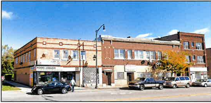
Left to right: 523 Lake Street, Maywood Motors Building and the Sanders Building in 2024.
