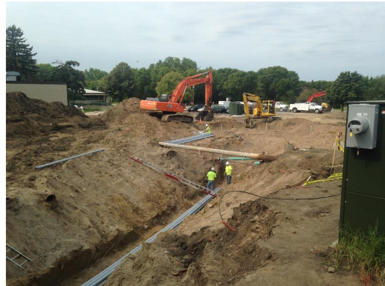
08/27/15 Installing the new underground electrical service below the existing electrical service being supported by the horizontal pole.
